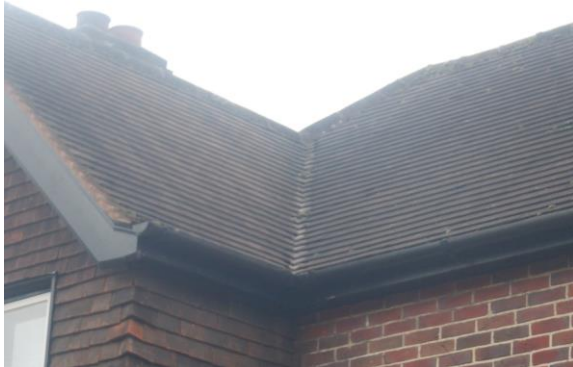
Photograph 3. Closely fitted roof tiles (front elevation).
