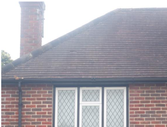
Photograph 5. Intact hip and ridge mortar.
