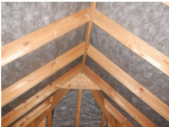
Photograph 12. Cobwebbed ridge; intact breathable membrane (roof void).
