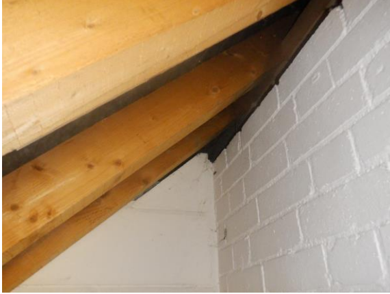
Photograph 17. Blockwork front gable (garage loft).
