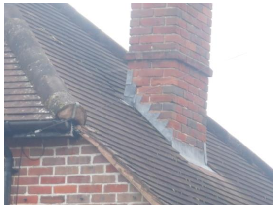
Photograph 9. Tight lead flashing around chimney (southern elevation).
