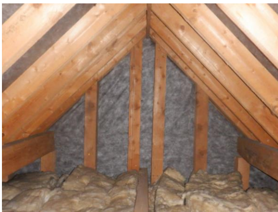
Photograph 15. Breathable membrane on the front gable end (roof void).
