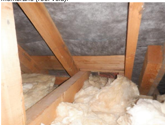
Photograph 14. Tight timber boarding around chimney at the eaves (roof void).
