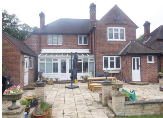
Photograph 2. Rear of property viewed from the east.
