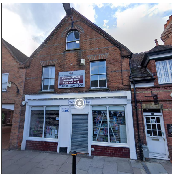
Figure 1 – Existing front Elevation of application premises.
