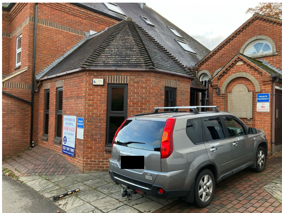
Picture 2: Three quarters view of the front/side elevations
