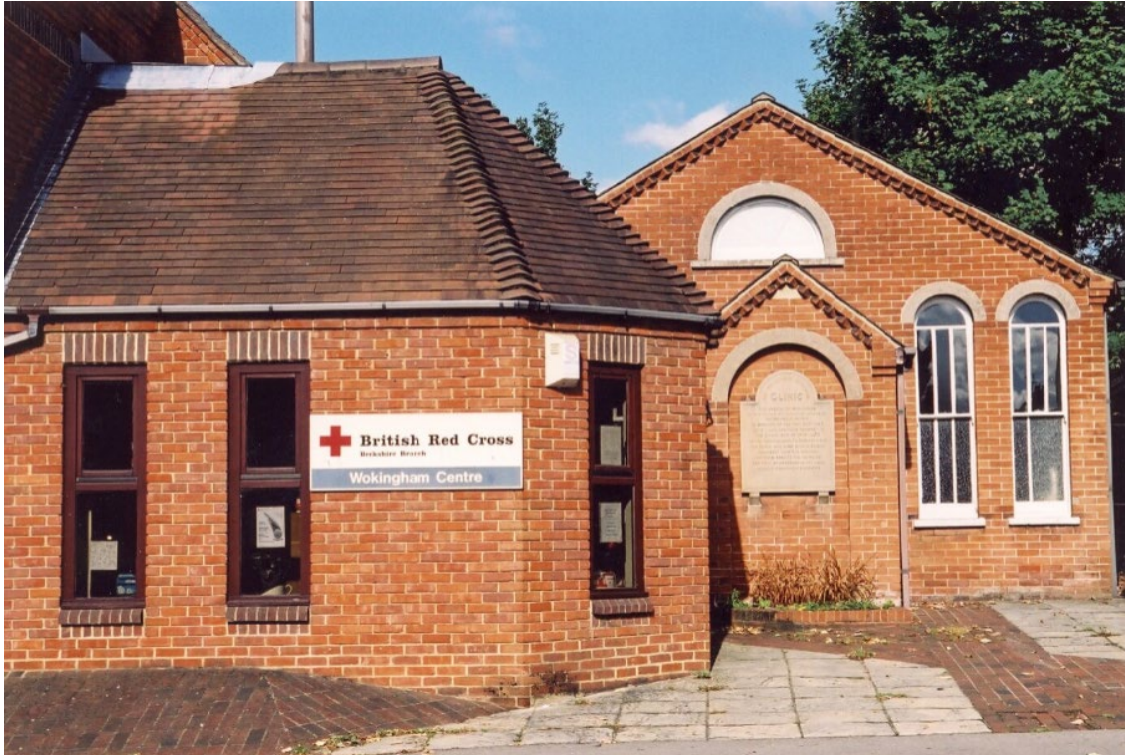
Picture 1: Front Elevations. Note the Existing Memorial Plaque centred on the porch.
