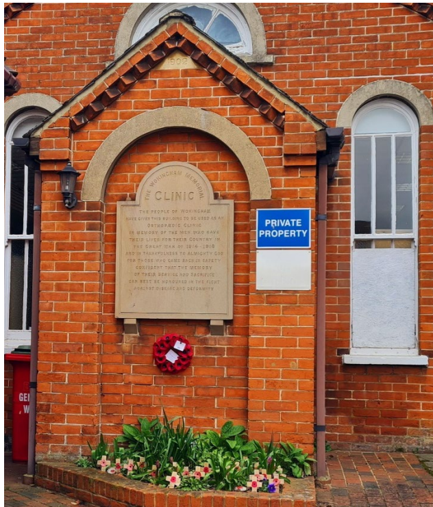
Picture 3: Close up of the Memorial Plaque (presently not illuminated)
