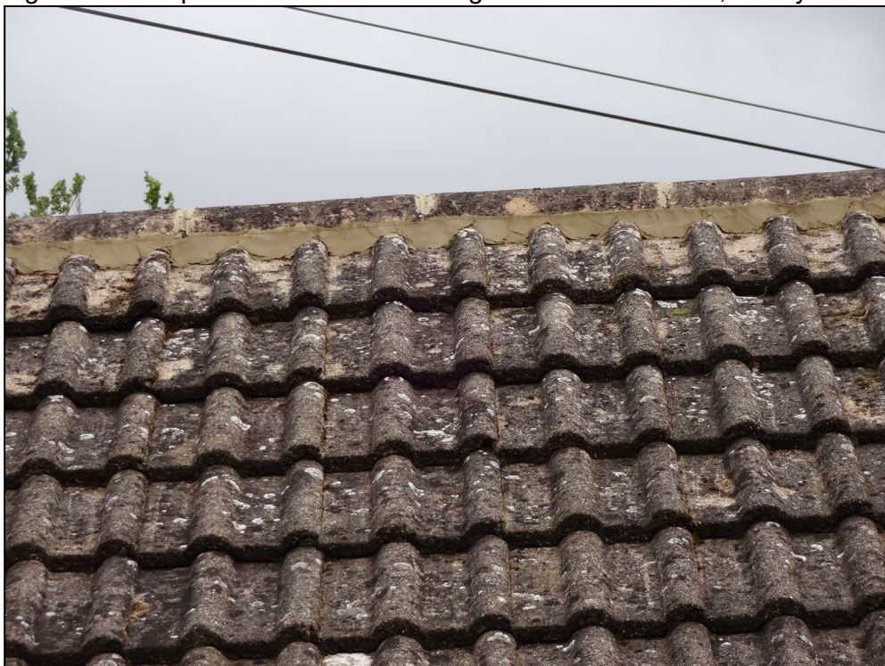
Figure 4. Example of sealed roof and ridge tiles. 33 Pitts Lane, Earley. 03.06.25
