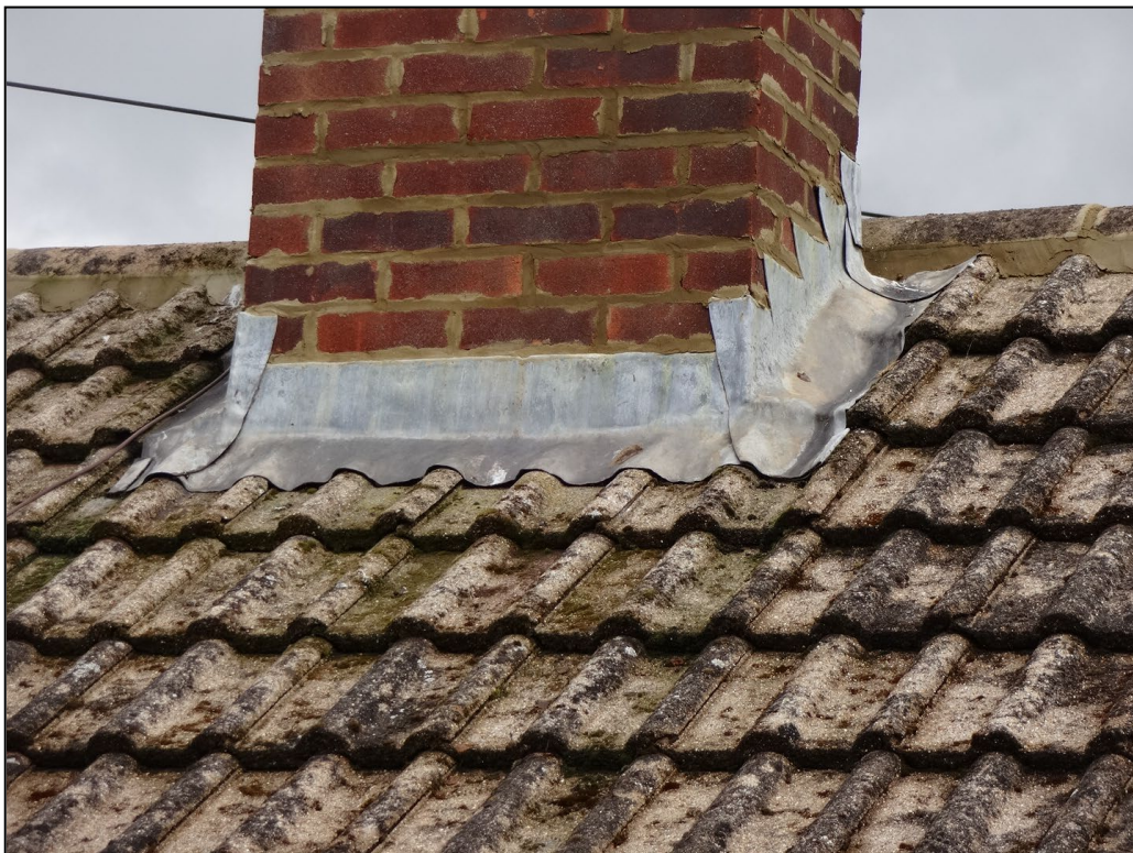
Figure 6. Example sealed lead flashing around chimney stack. 33 Pitts Lane, Earley. 03.06.25
