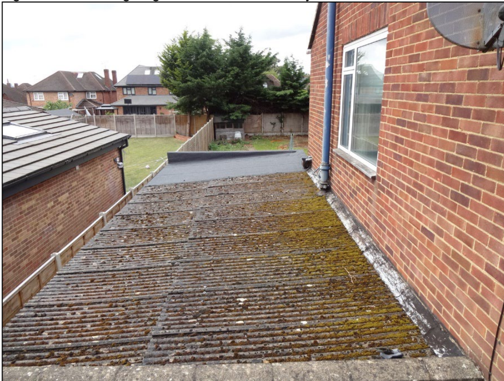
Figure 10. Roof of garage. 33 Pitts Lane, Earley. 03.06.25
