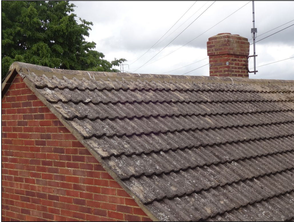
Figure 5. Example of sealed verges. 33 Pitts Lane, Earley. 03.06.25
