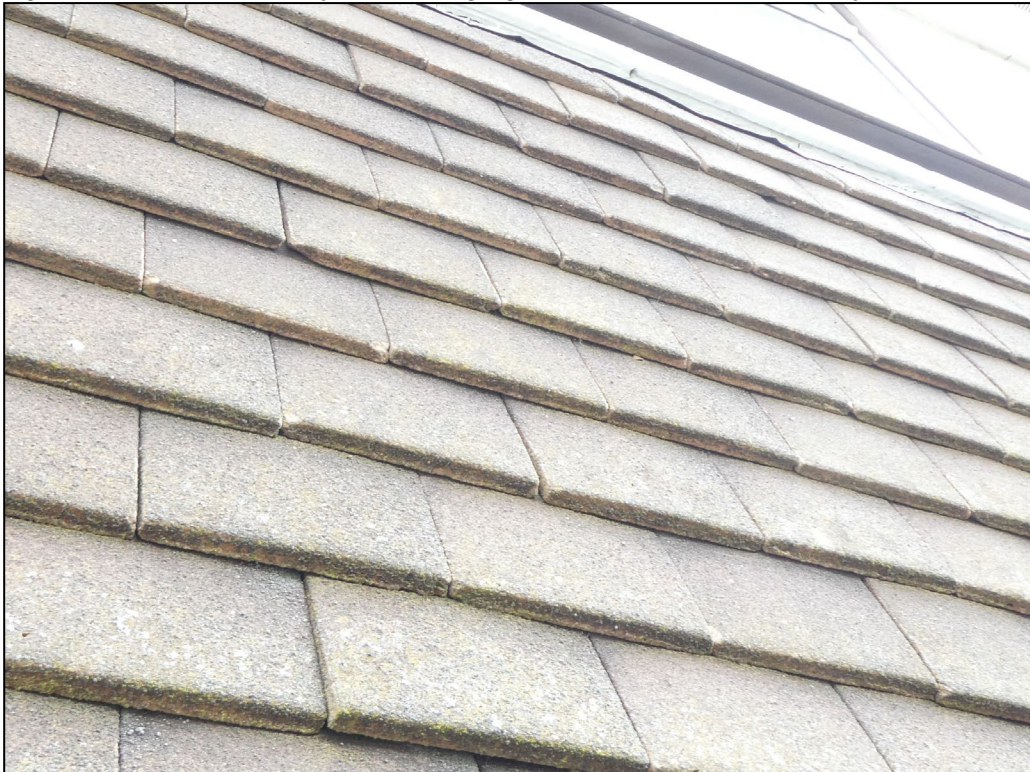
Figure 8. Example closely fitted hanging tiles. 33 Pitts Lane, Earley. 03.06.25
