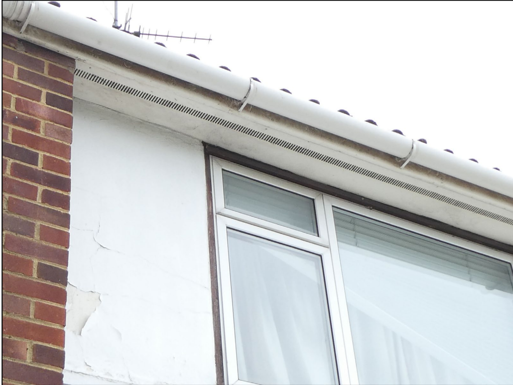
Figure 7. Example sealed uPVC soffits/fascias. 33 Pitts Lane, Earley. 03.06.25
