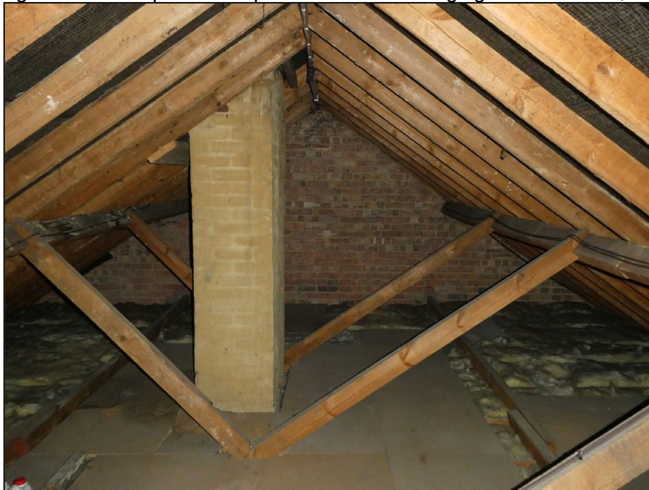
Figure 13. Example of loft space and bitumen lining. 33 Pitts Lane, Earley. 03.06.25
