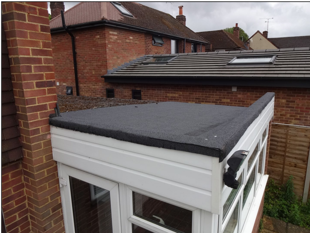
Figure 12. Example sealed roof and fascias on summer room. 33 Pitts Lane, Earley. 03.06.25
