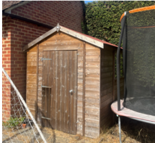
Building B3, southern elevation
