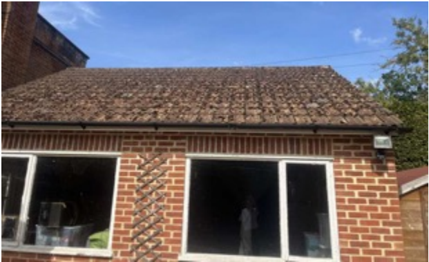
Building B2, southern elevation
