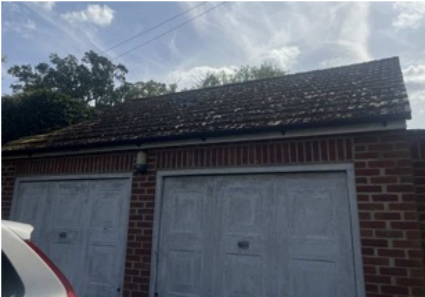
Building B2, northern elevation
