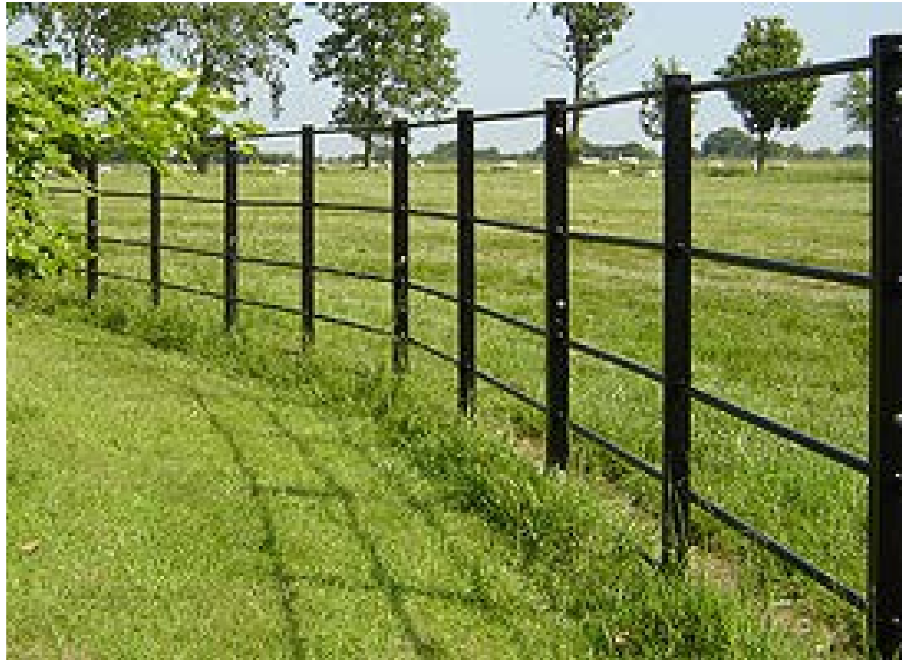
Metal estate railings
