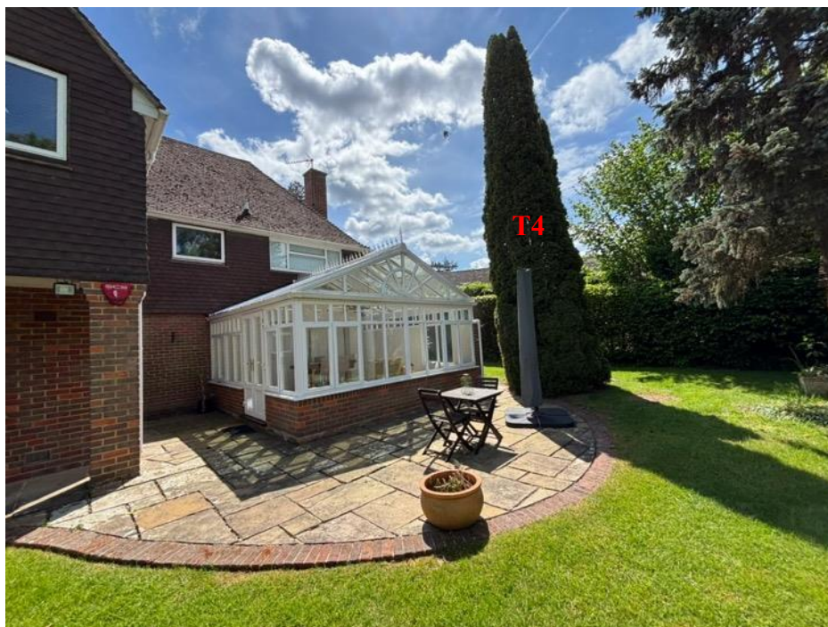
Photoview 8: View looking south at T4.
