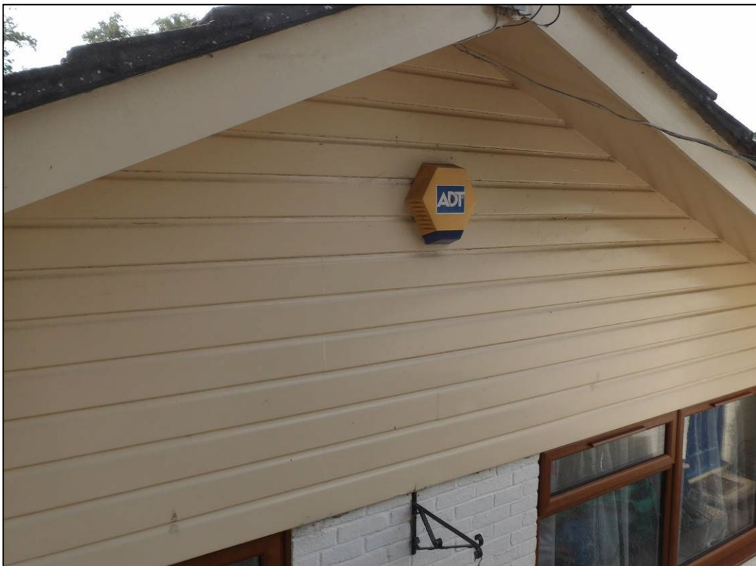
Figure 8. Tightly fitted wooden cladding. Beamis Lodge, Fleet Hill, Finchampstead, 27.08.24
