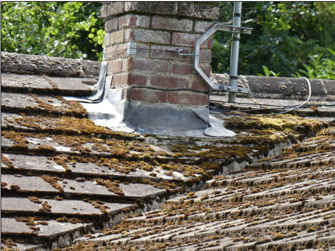
Figure 6. Lead flashing around the chimney. Beamis Lodge, Fleet Hill, Finchampstead, 27.08.24
