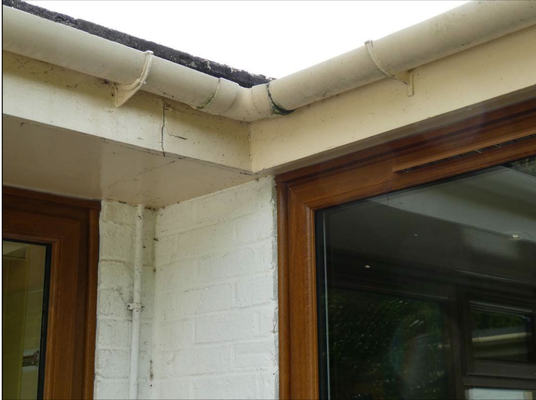
Figure 7. Example of soffits and fascias. Beamis Lodge, Fleet Hill, Finchampstead, 27.08.24
