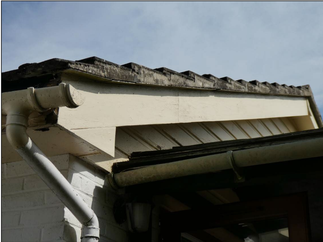
Figure 5. Example of verges. Beamis Lodge, Fleet Hill, Finchampstead, 27.08.24
