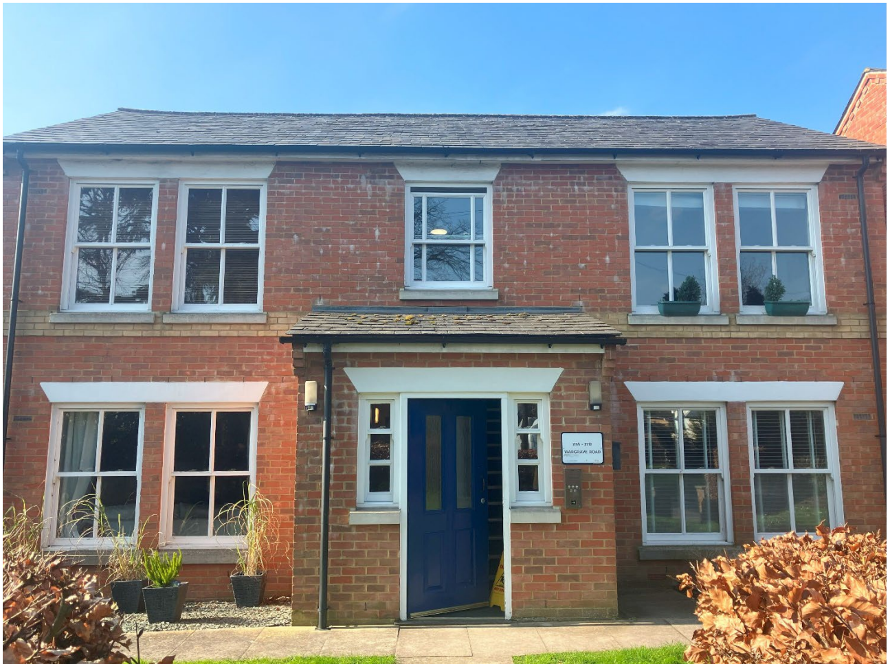
Figure 1 - Front elevation of property
