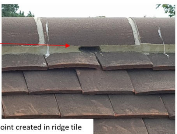
Example of a single access point created at gable end
