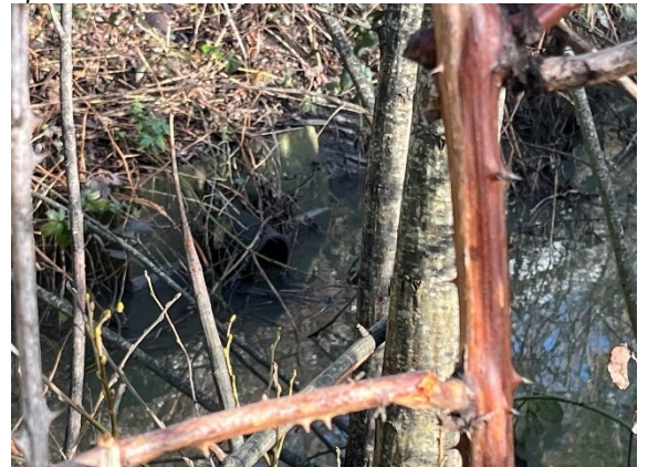
Photograph 8. Pipe on the northern bank of the river.
