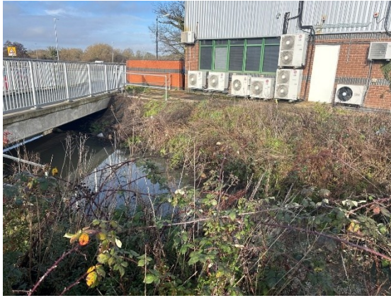
Photograph 3. Western end of the site viewing the northern bank.
