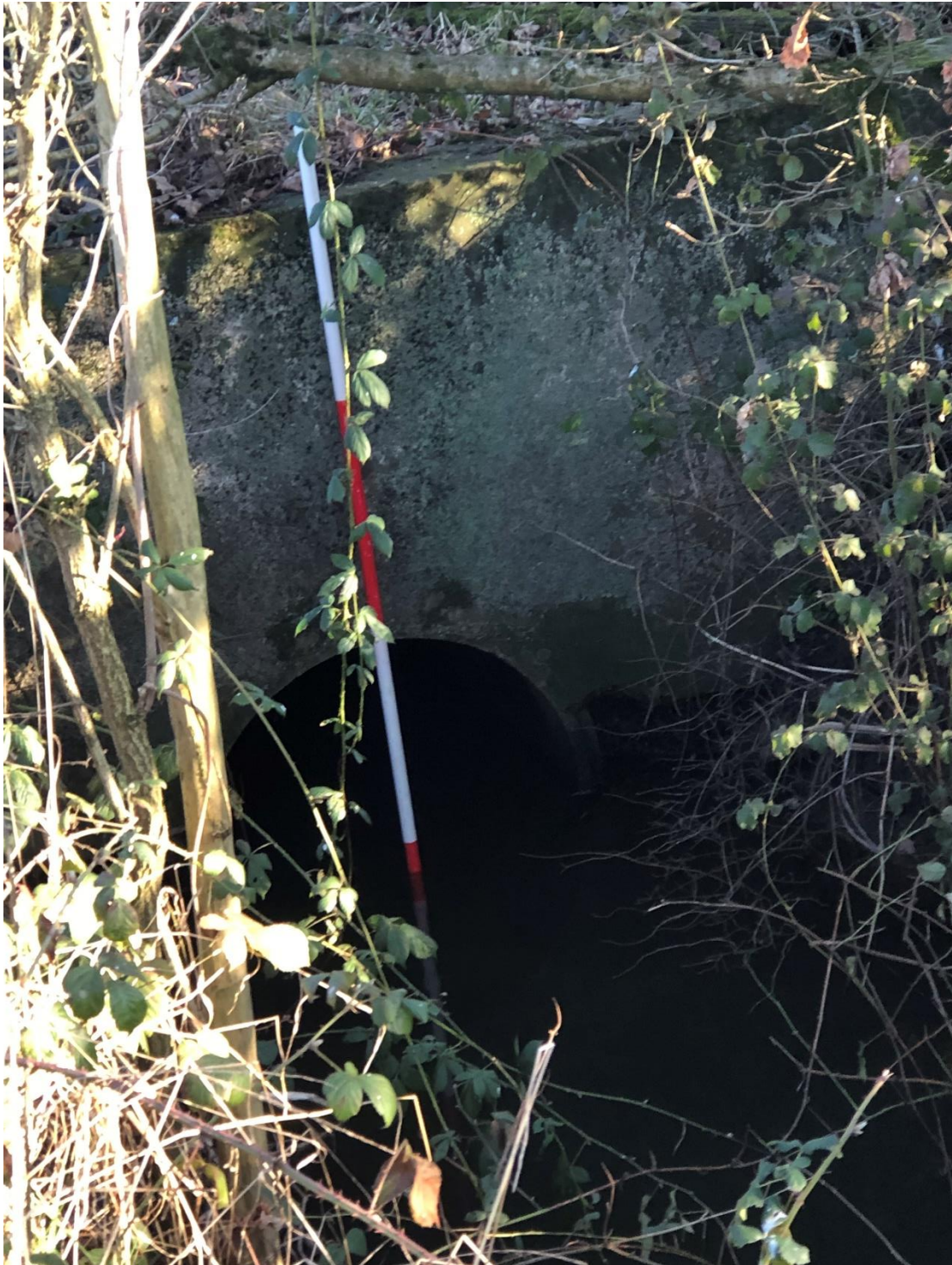
Figure 7 – Ordinary Watercourse Central Crossing
