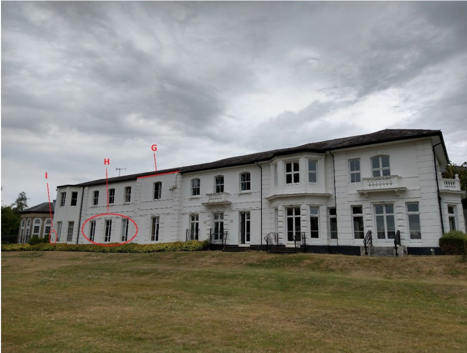
Photograph 3: South western elevation of B2 with the lounge (B3), adjacent. Showing location of features G (gap along eaves), H (small recesses around window frames) and I (vertical crack in stonework).
