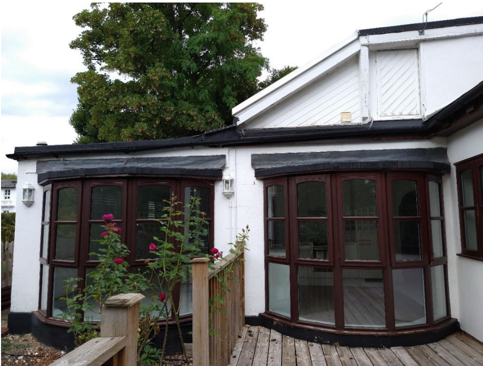
Photograph 8: South eastern elevation of B6 with bay windows
