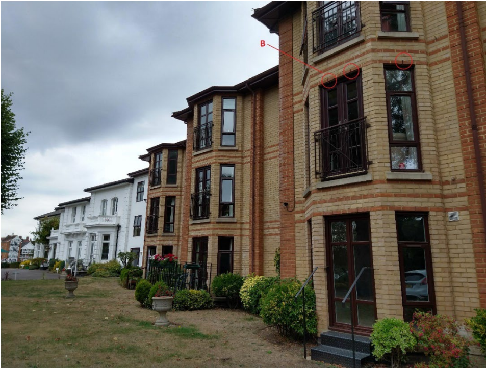
Photograph 1: South eastern elevation of B1, showing weep holes present above first floor windows (Feature B). Weep holes were also present over windows / doors on the ground floor.
