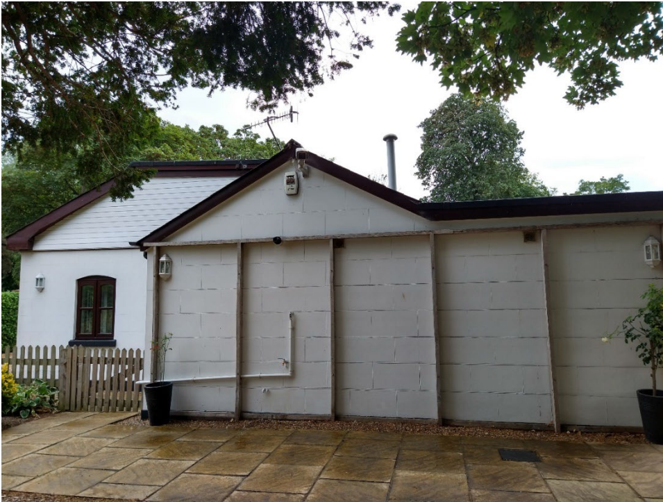
Photograph 9: North western elevation of B6
