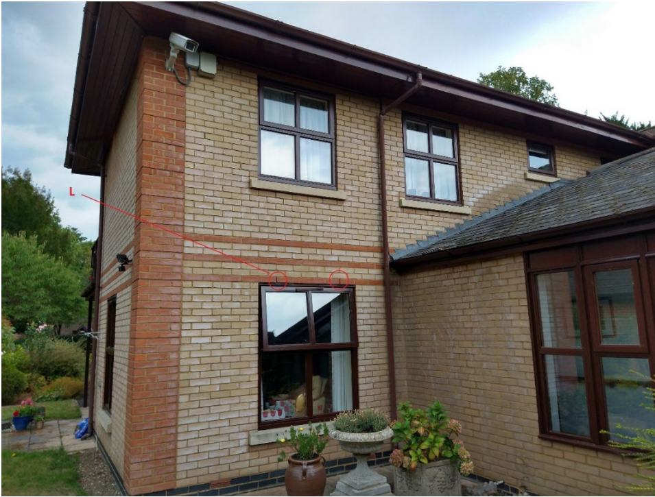
Photograph 7: Section of B5 showing weep holes (Feature L) above ground floor windows.
