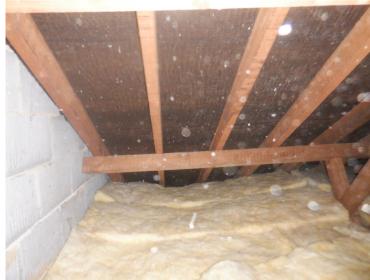
Photograph 19. Thick fiberglass insulation and no gaps in brick work.
