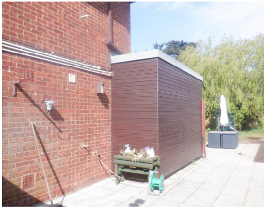
Photograph 17. North-east rear extension tightly fitted to brick wall of main building.
