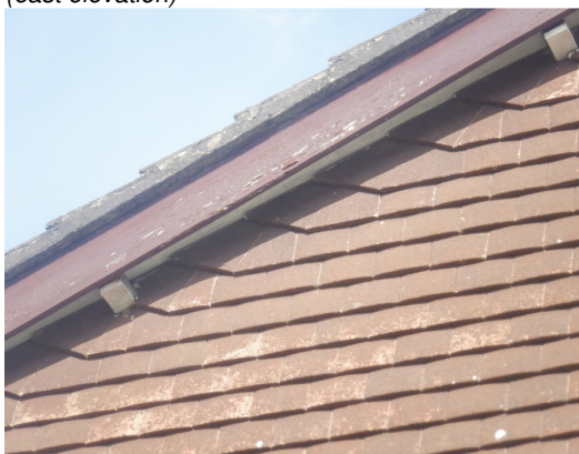
Photograph 11. Intact verge mortar (south elevation)
