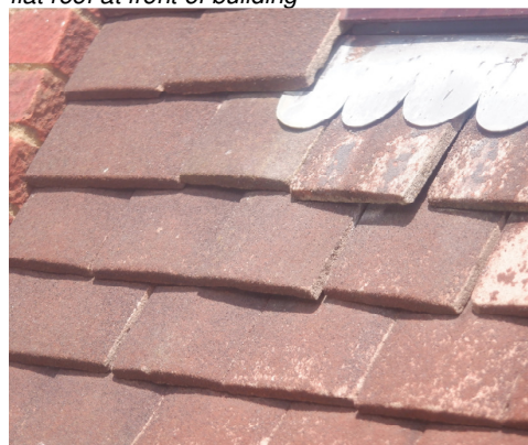
Photograph 7. Gaps at the bottom of the front
