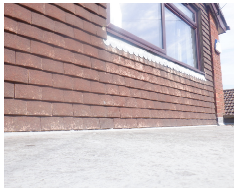
Photograph 5. Hanging tiles tight at the base to flat roof at front of building
