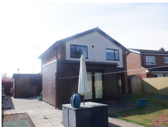
Photograph 3. Garage and existing rear extension attached to the eastern and northern sides of the house.
