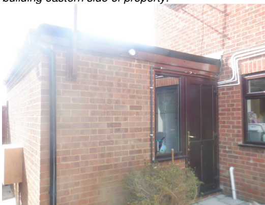
Photograph 14. Garage flat roof with tight bitumen roofing felt.
