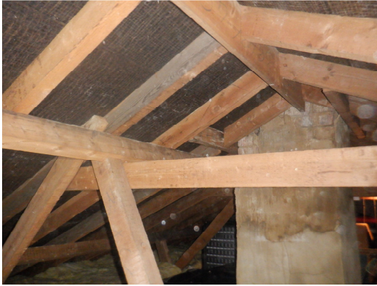
Photograph 18. Tight/intact bitumen felting across whole loft void with no tears.
