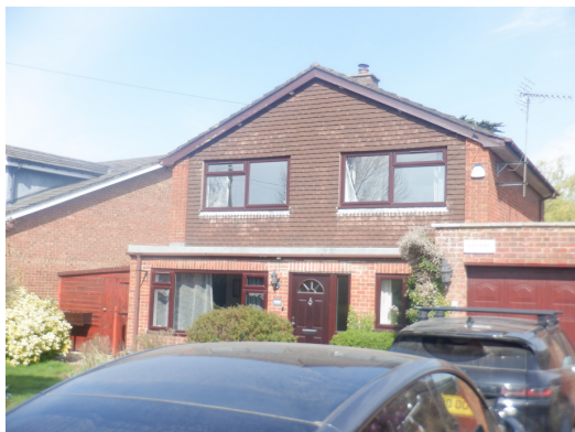
Photograph 1. Front of the house viewed from the south.
