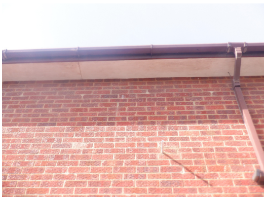
Photograph 9. Soffit boxes tight to the brickwork (east elevation)
