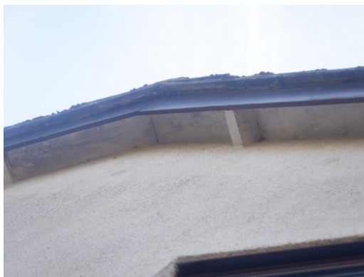
Photograph 10. Soffit boxes tight to rear (north facing) rendered wall and fascias intact
