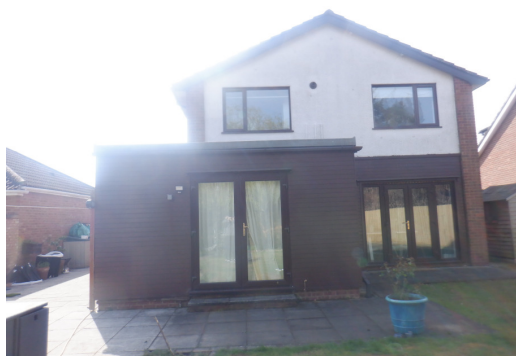
Photograph 2. Rear of the house viewed from the north.
