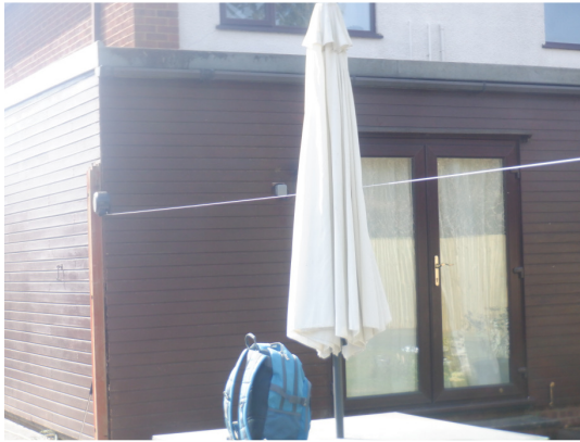
Photograph 16. Existing rear extension.
