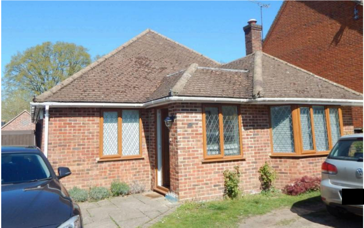
Image 1 – South facing elevation of the property
