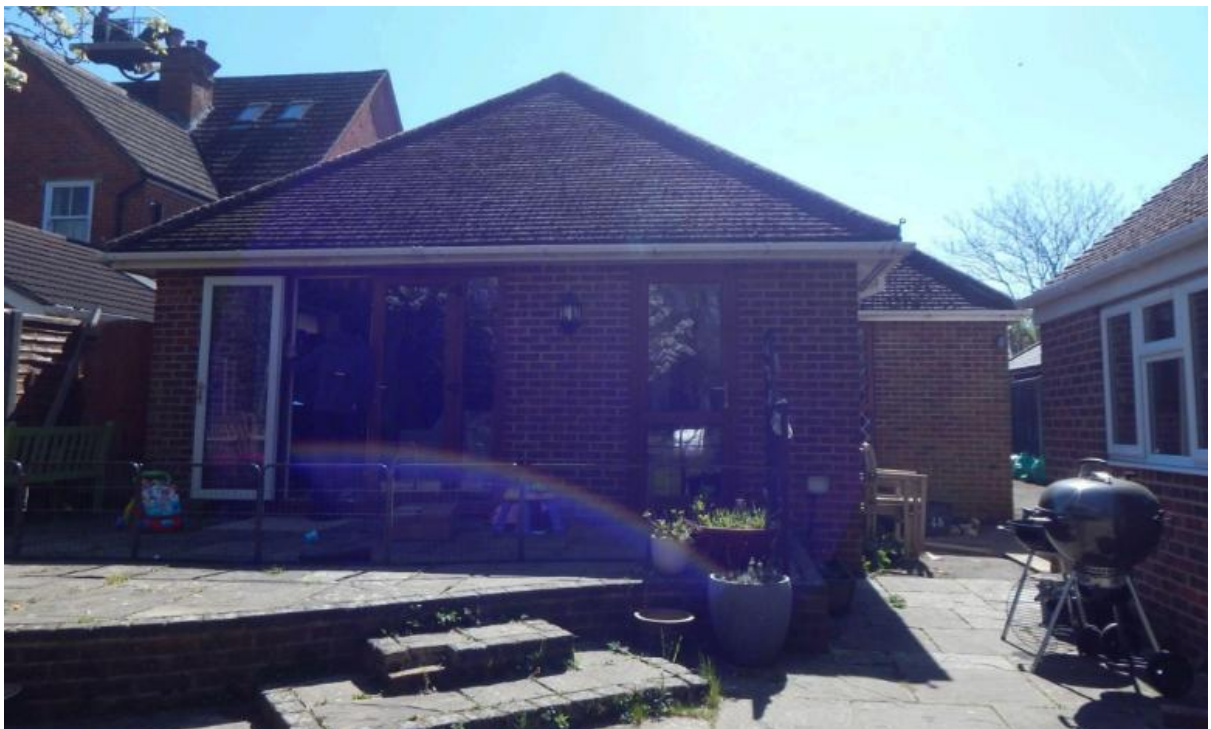
Image 4 – North facing elevation of the property
