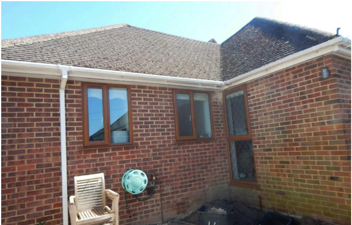
Image 2 – West facing elevation of the property
