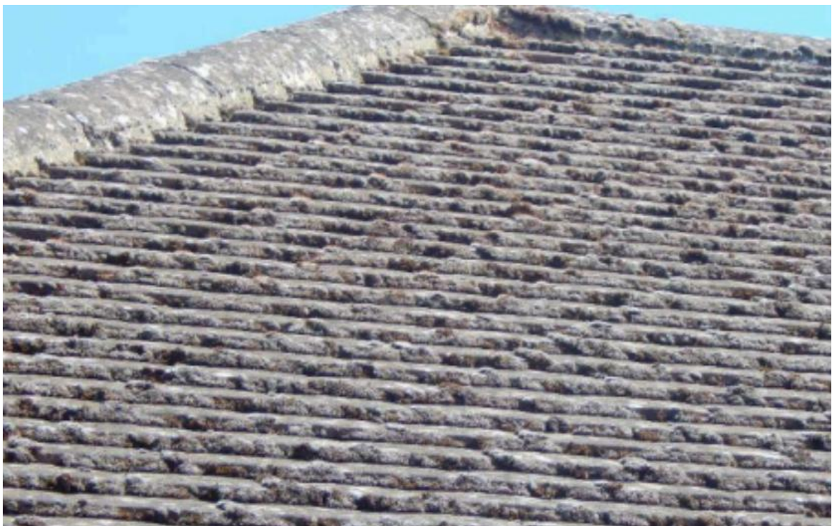
Image 6 – Example image of the main tiled roof coverings to demonstrate condition
