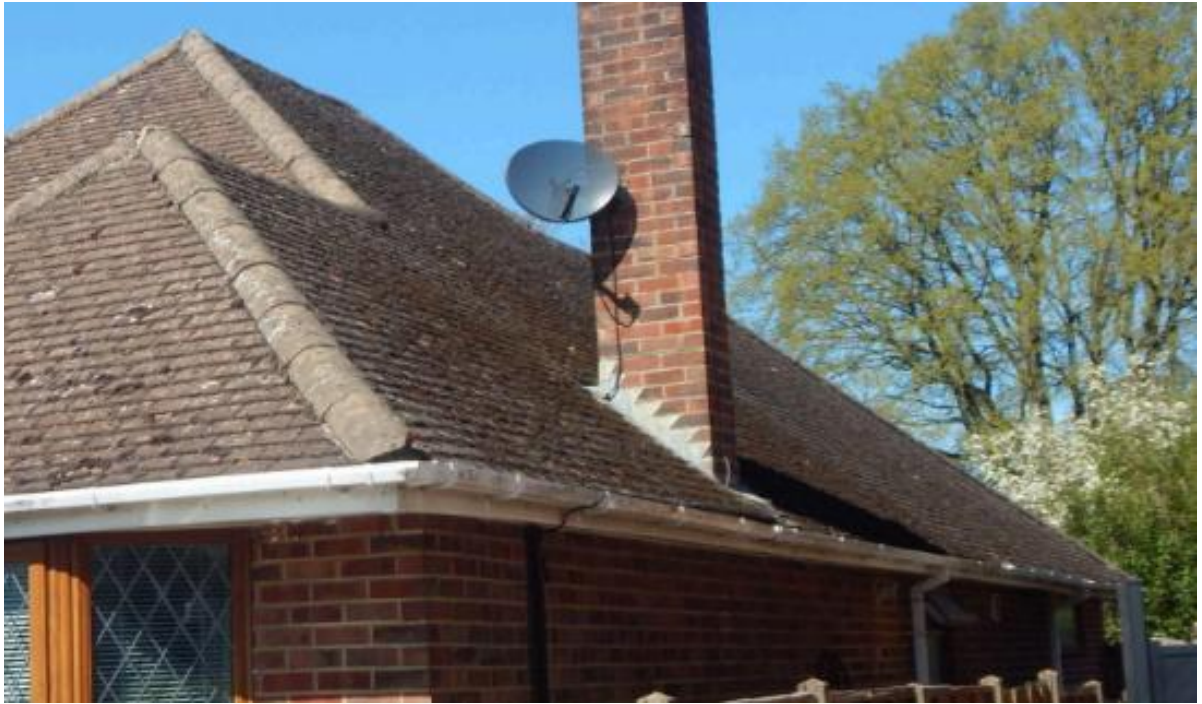
Image 3 – East facing elevation of the property
