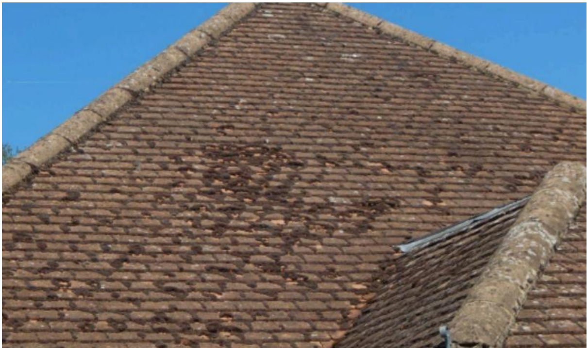
Image 5 – Example image of the main tiled roof coverings to demonstrate condition
