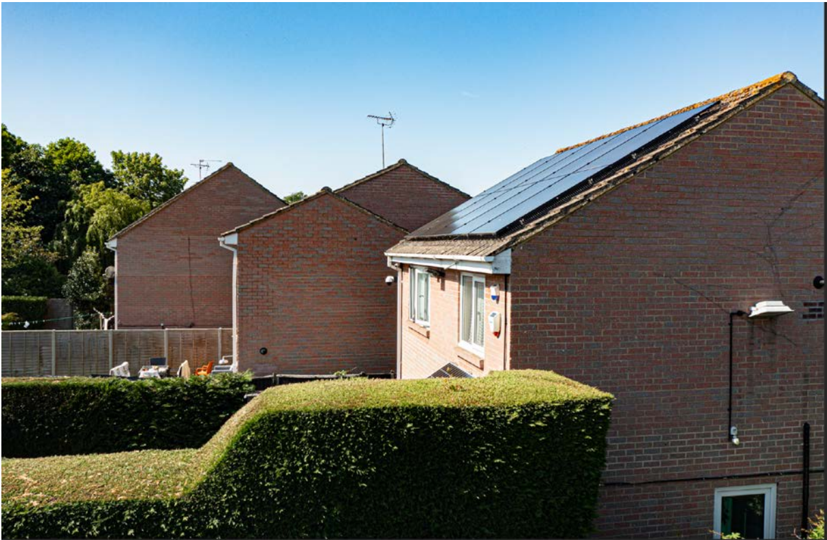
After: - Shadowing to Solar Panels and Living Spaces (Lounge , Bedroom, Kitchen)
