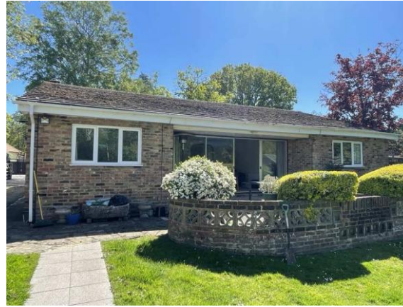
Western elevation of B1
