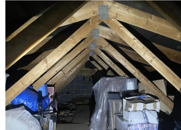
Loft space within B1
