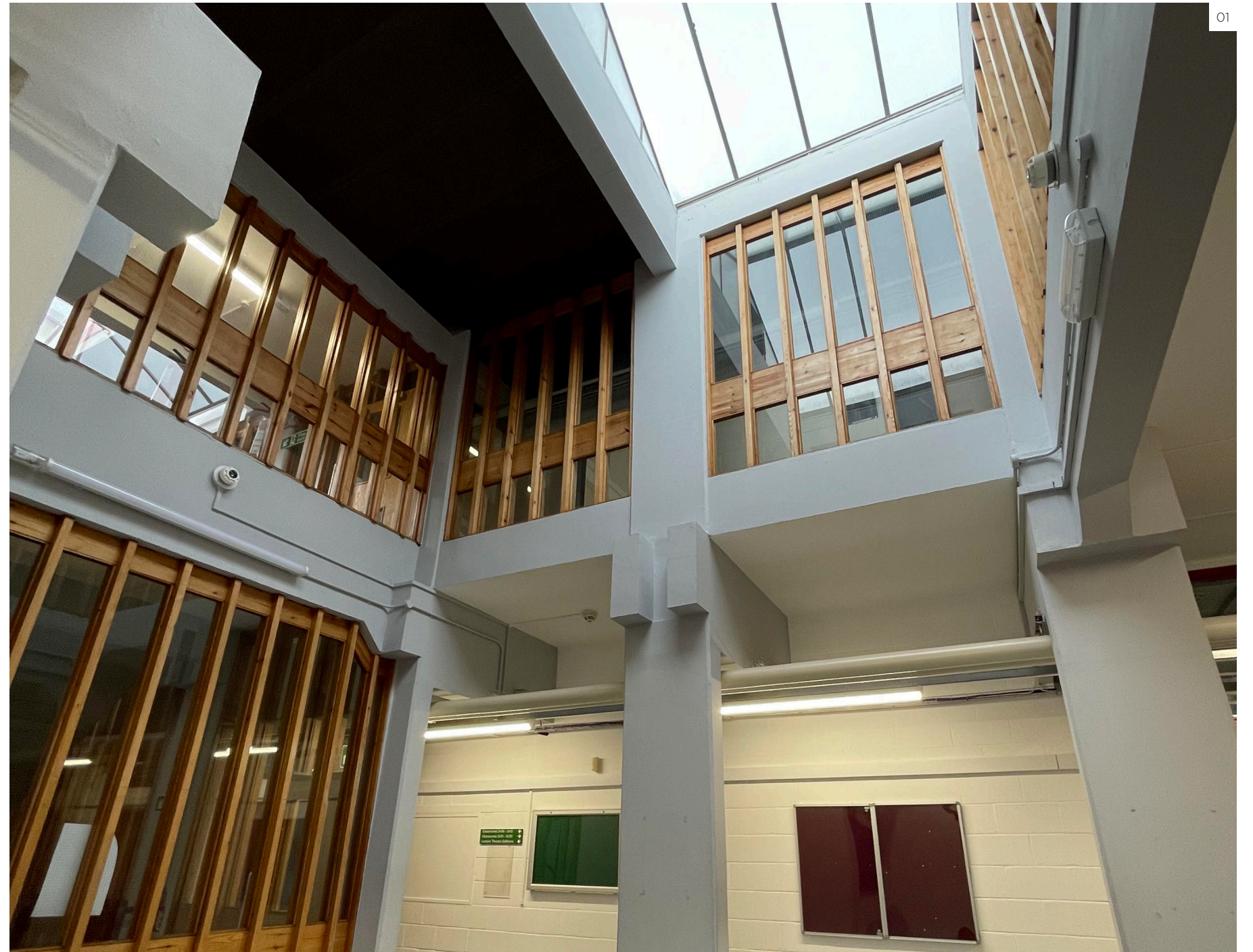
01 Photo of existing second floor timber screen lightwell.
