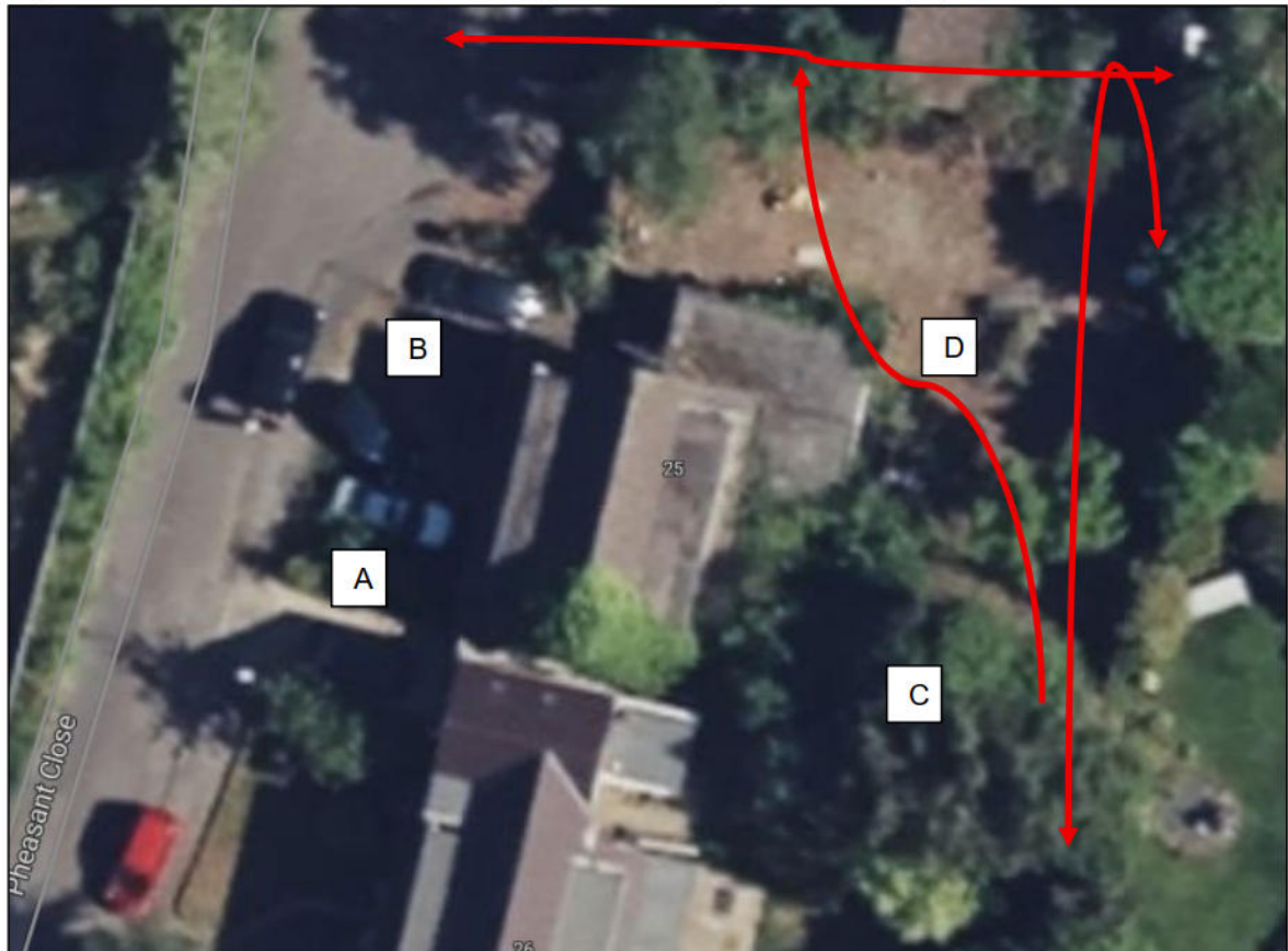
Figure 1 – 25 Pheasant Close, Wokingham, surveyor/remote equipment locations.
