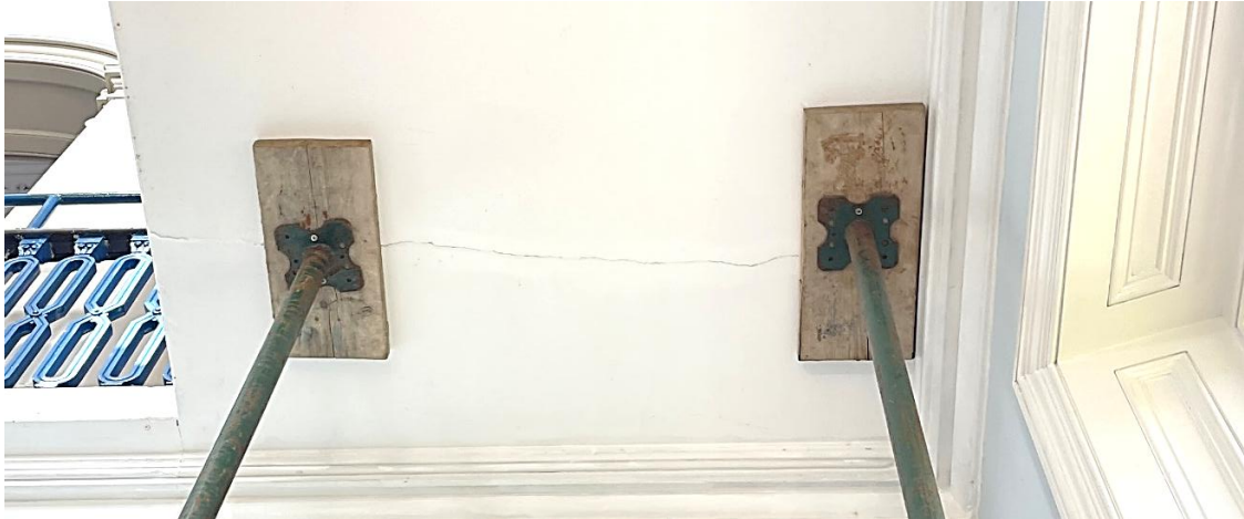
Figure 3. The cracking to the first floor landing – underside.
