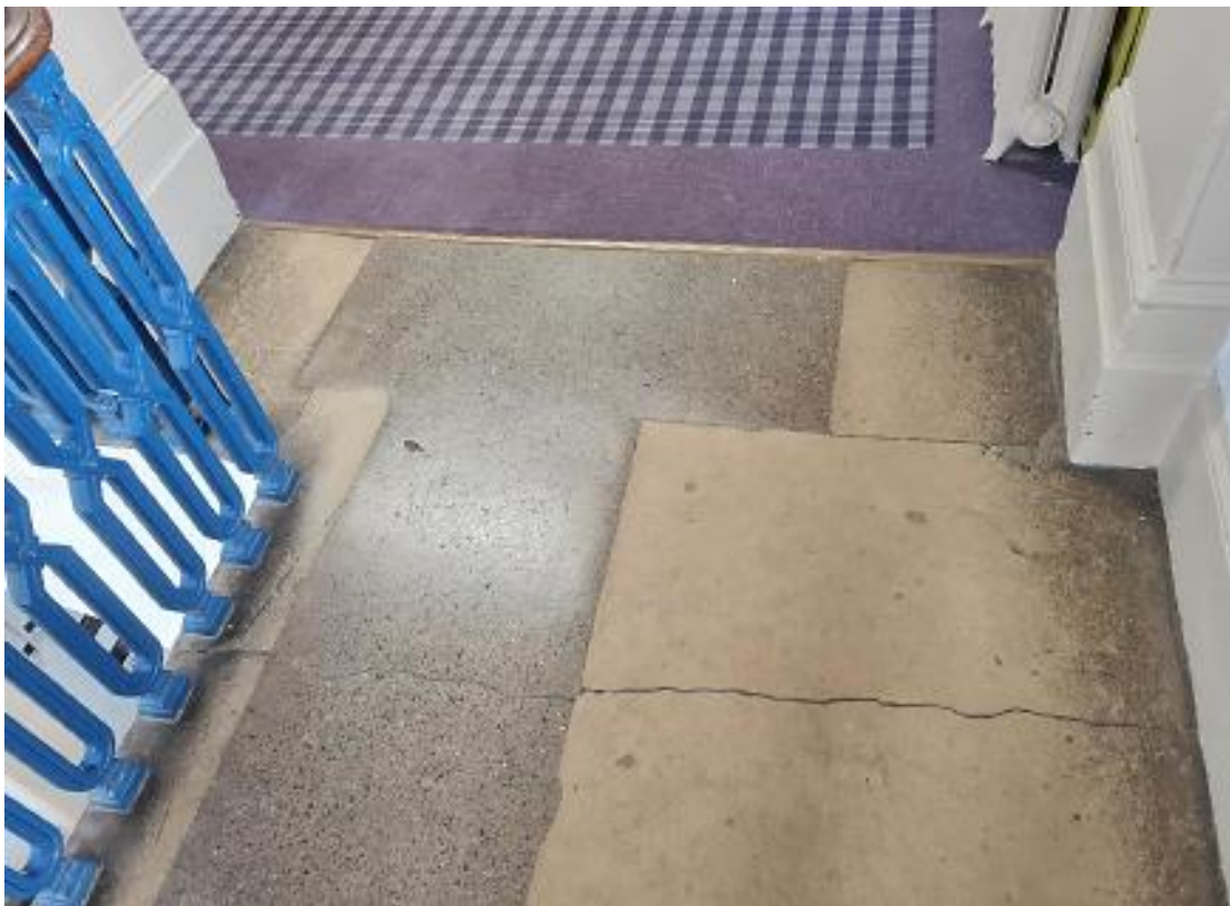
Figure 4. The cracking in the first floor landing.
