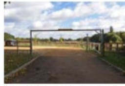
Height restricting barriers to car park entrance with retractable swinging across gate and open locking post
