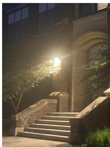
Poor high glare wall light
