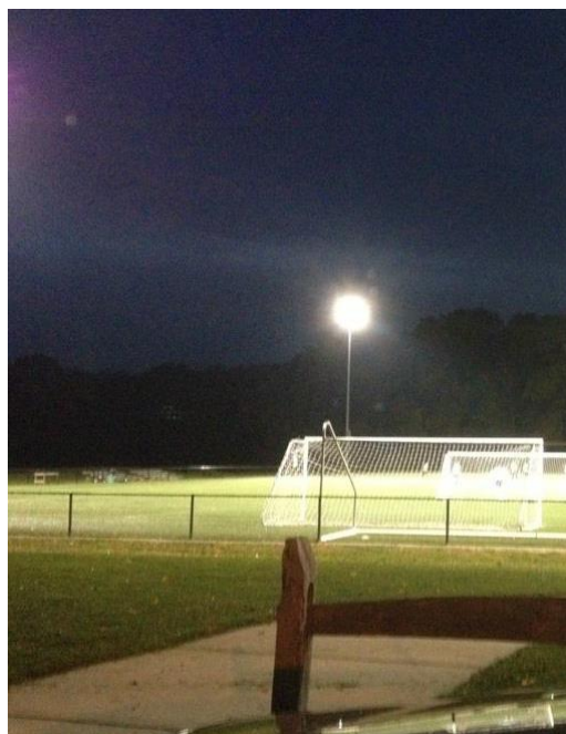
Low quality flood lighting
