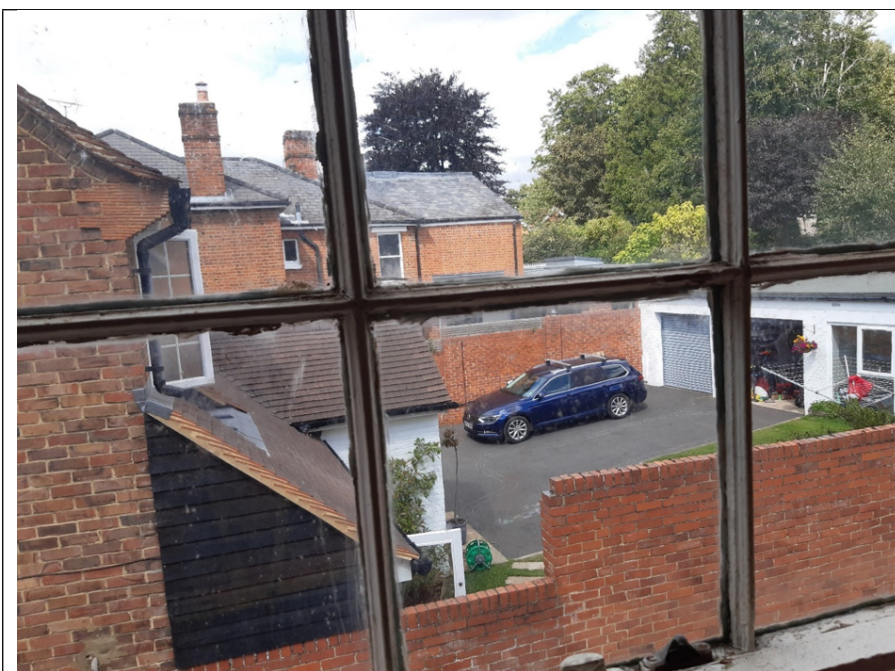
Fig. 3: First floor north facing window looking towards rear of 41 High Street
