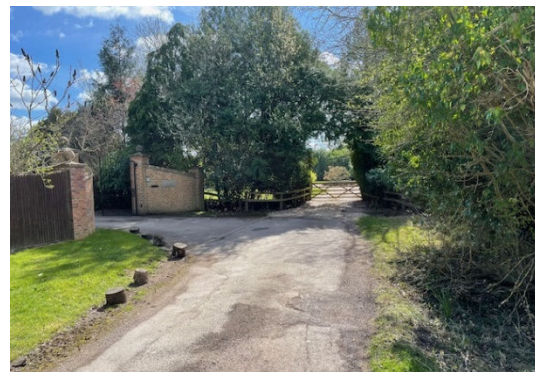
Gates and walls/fencing to adjoining houses
