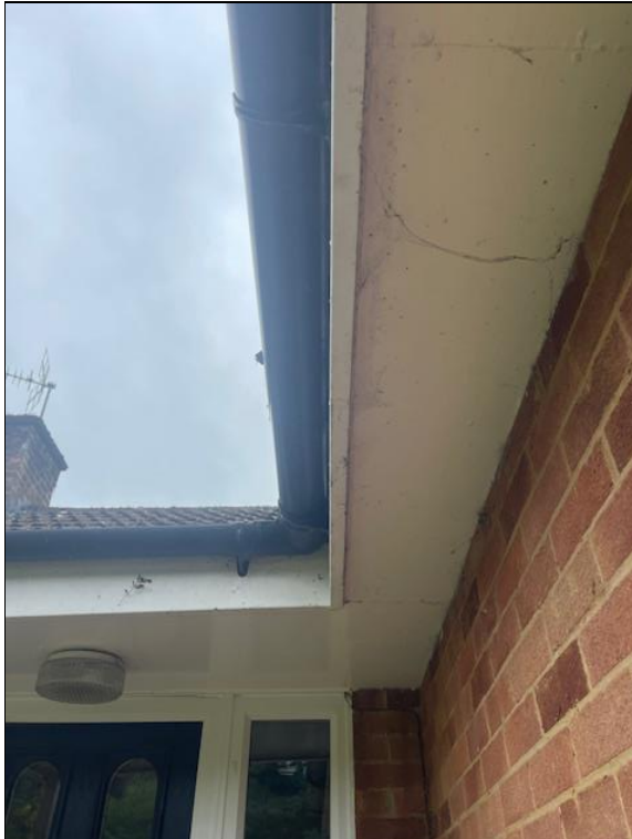
Photograph 5: Wooden soffits in good condition.
