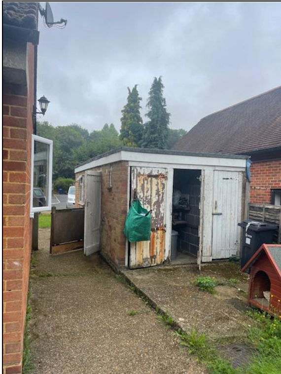
Photograph 17: Adjacent flat-roofed shed.
