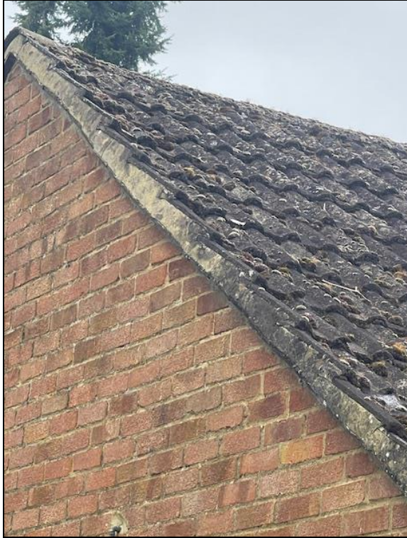
Photograph 11: No gaps around roof tiles, cemented sides.
