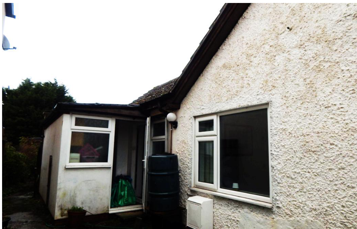
Image 5 – West facing elevation of the property
