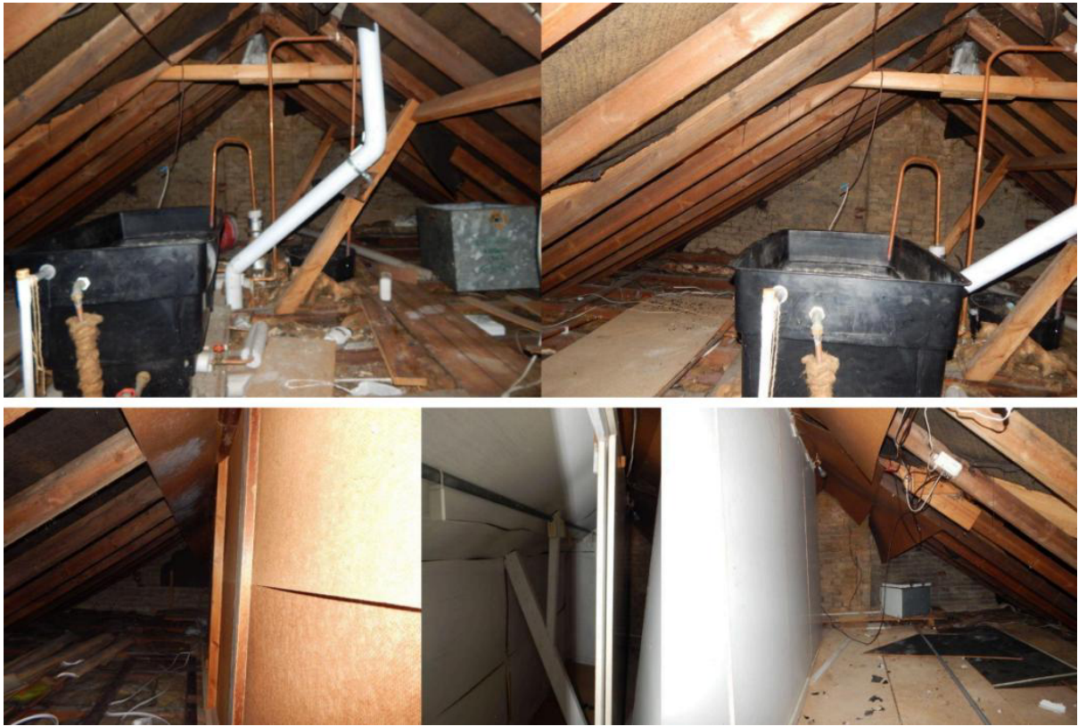
Image 7 – Internal views from within the main roof void spaces of the property
