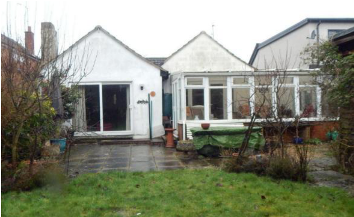
Image 3 – North facing elevation of the property
