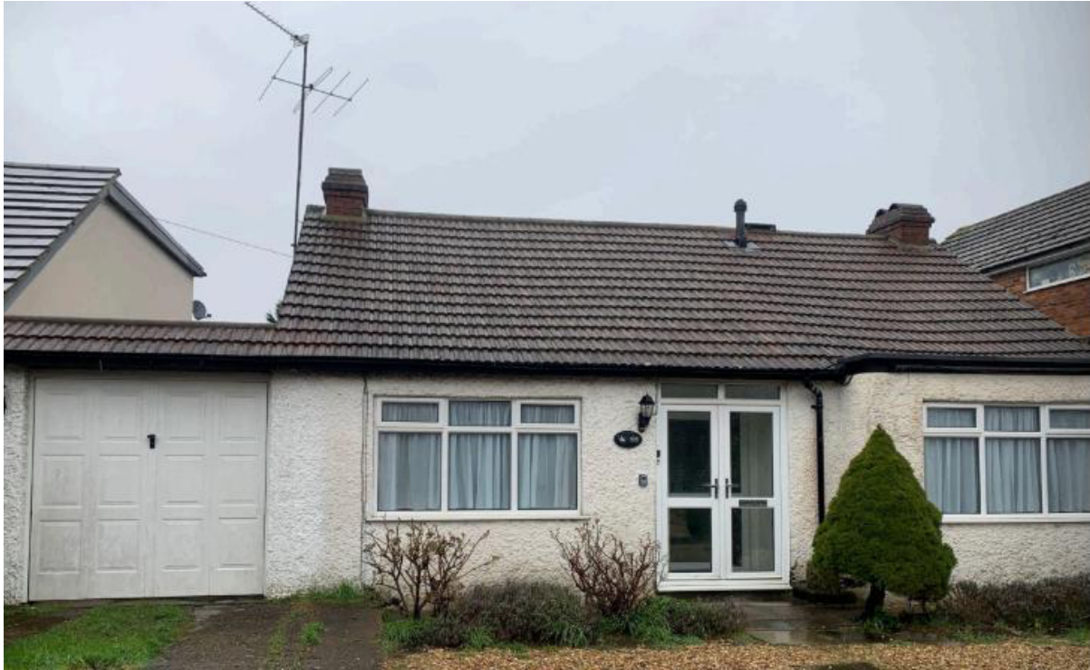
Image 1 – South facing elevation of the property
