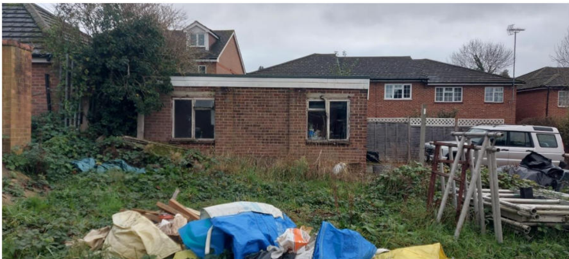
Plate 2. Existing garage to the southeast of the Site.
