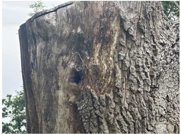
T12 close up of rot hole
