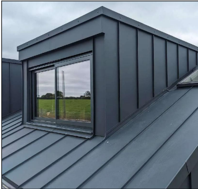
Standing Seam Metal Roof
