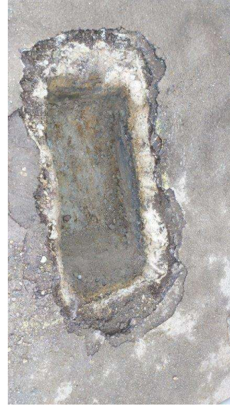
Photograph 8 - Looking down at TP02.
