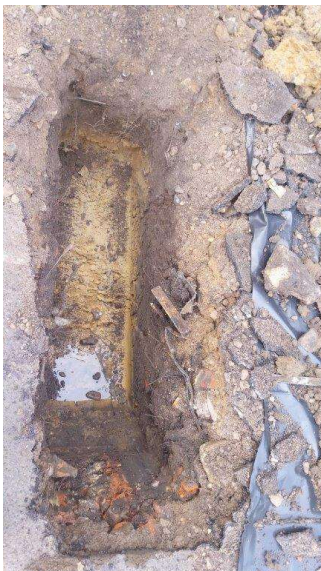
Photograph 5 - Looking down at water seepage encountered at 0.8m bgl within TP01.
