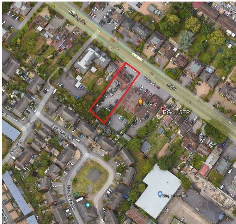
Figure 1: Site Location. Site Location. (Map data ©2023 Google)
