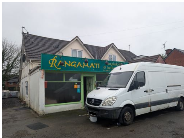
Image 8: Northern elevation of the building on site, facing southwest
