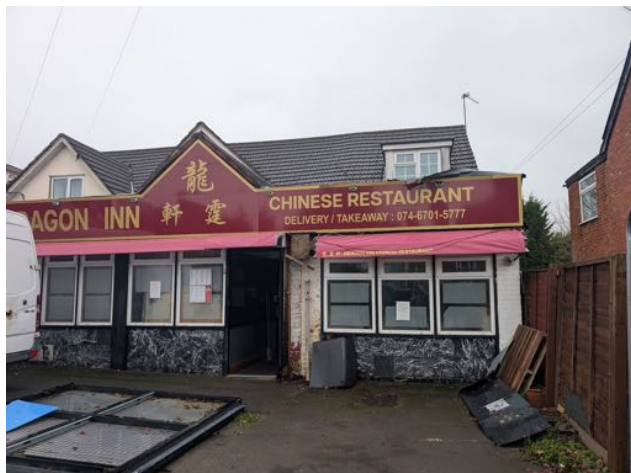
Image 7: Northern elevation of the building on site, facing south
