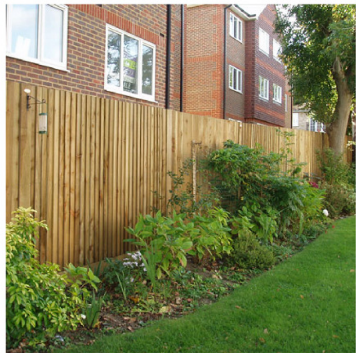
close boarded fence (1.8 or 2m where shown)
