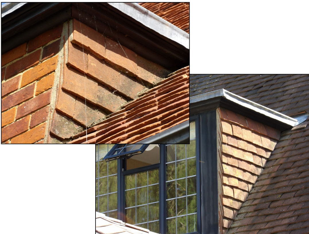
Figure 10. Example sealed verges and hanging tiles on dormer windows. Coombe Hill, Barkham. 29.04.25
