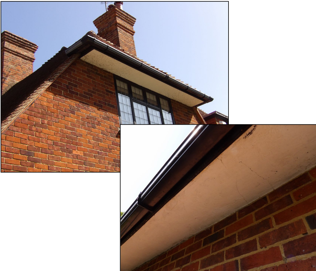
Figure 8. Example sealed soffits and fascias. Coombe Hill, Barkham. 29.04.25
