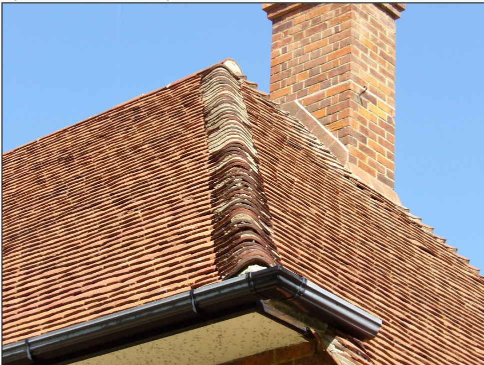
Figure 6. Example missing mortar in bonnet tiles. Coombe Hill, Barkham. 29.04.25
