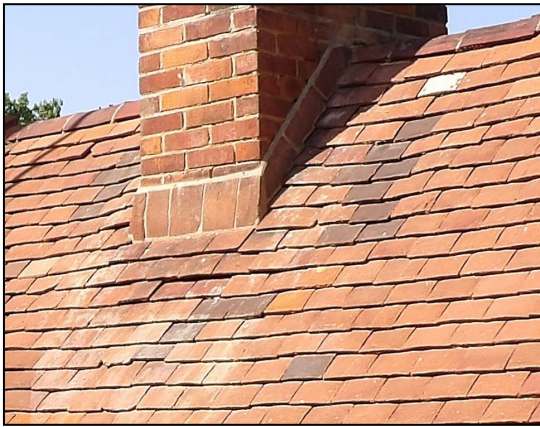
Figure 6. Example missing mortar in bonnet tiles. Coombe Hill, Barkham. 29.04.25
