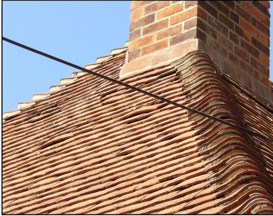
Figure 5. Example raised tiles near chimney stacks. Coombe Hill, Barkham. 29.04.25
