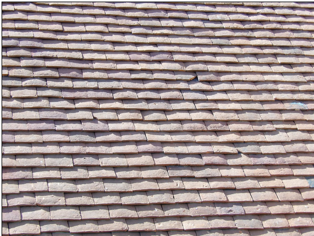
Figure 4. Examples roof tiles. Coombe Hill, Barkham. 29.04.25
