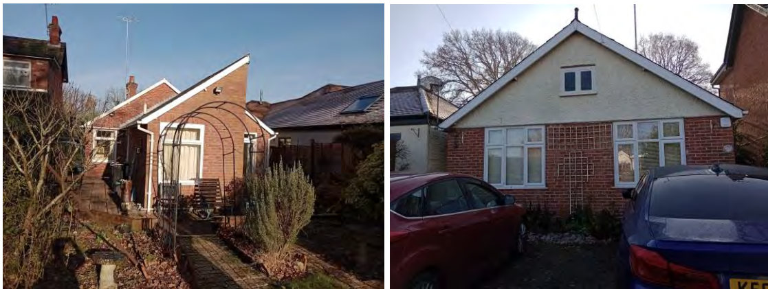
Figure 1 and 2: Front and rear elevation at 13 Ellis Road
