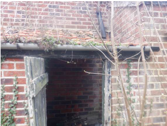
Photograph 9. Brick sheds (rear elevation).
