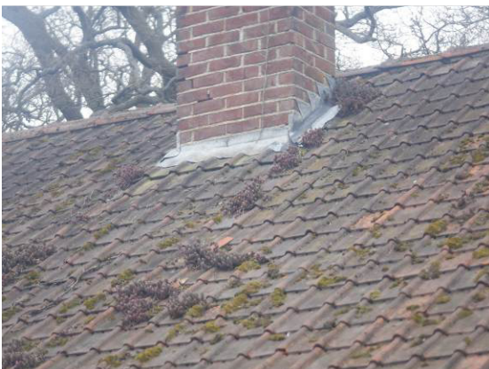
Photograph 5. Lead flashing flush around chimney (rear elevation).
