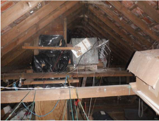
Photograph 11. Bungalow roof void.
