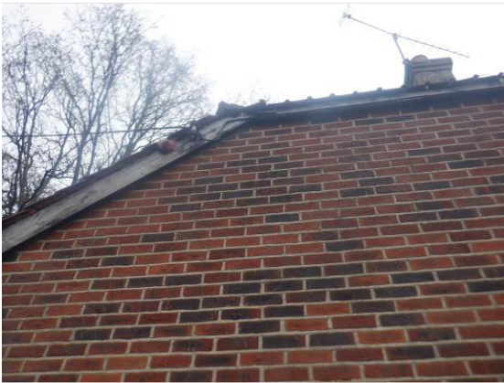
Photograph 7. Barge boards at half-hipped gables (southwest elevation).
