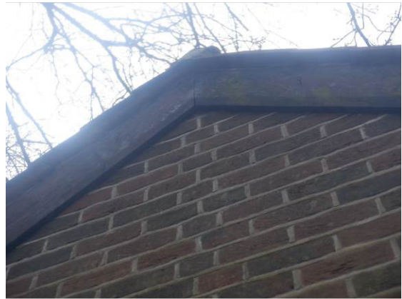
Photograph 8. Barge boards at front gable (front elevation).
