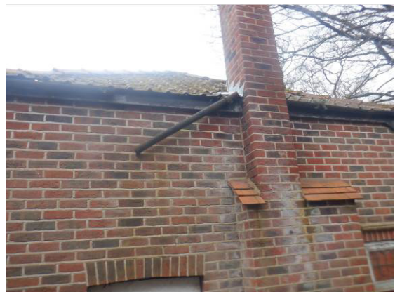
Photograph 6. Lead flashing flush around chimney (northeast elevation).
