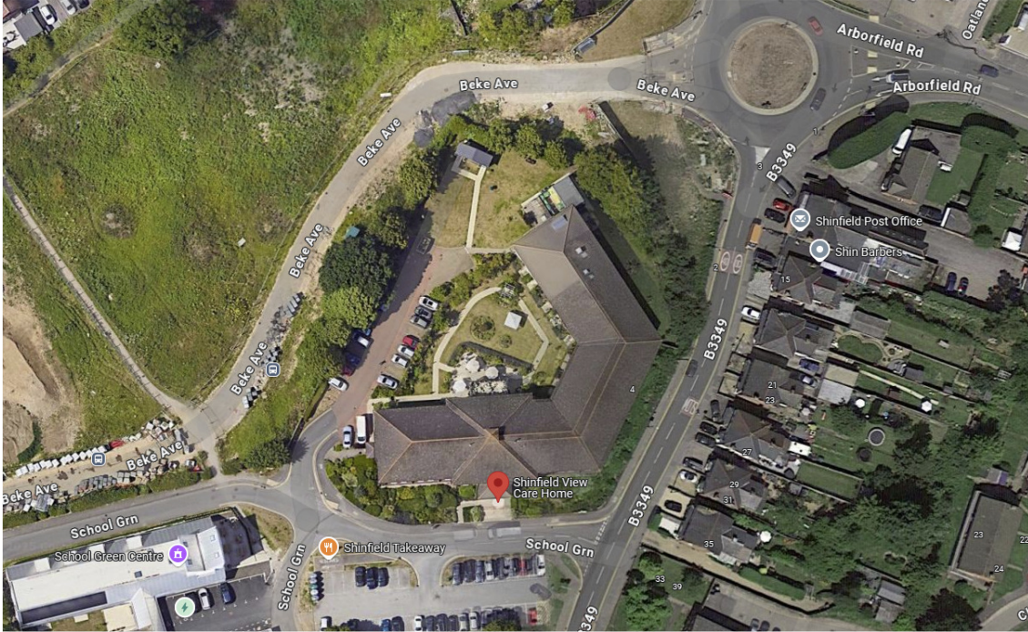
Figure 1: Aerial view of Shinfield View Care Home
