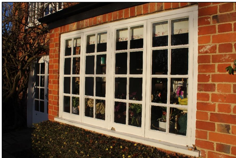
Photograph 2 – Kitchen window of rear extension likely built in the 1950s
