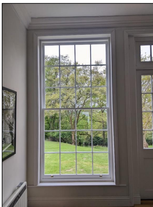
Photograph 4 – An example of the traditional timber, double glazed sashes installed
