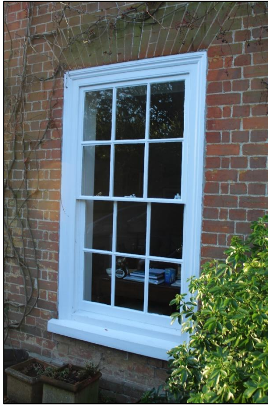
Photograph 1 – Typical six over six pane sash window on the ground floor of the original dwelling with the rebate infilled with a Georgian style architrave
