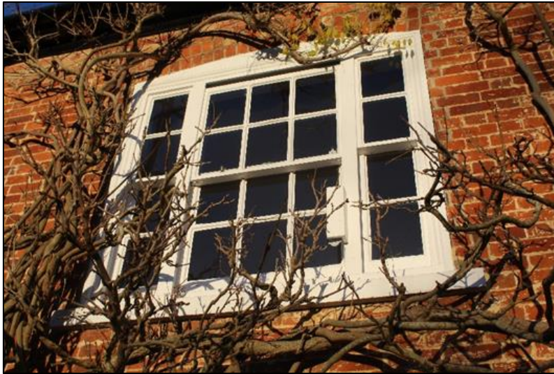
Photograph 3 – First-floor bedroom window to two-storey side extension with similar Georgian architrave to the exterior edge.
