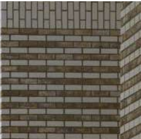
Contrasting brick band detailing
