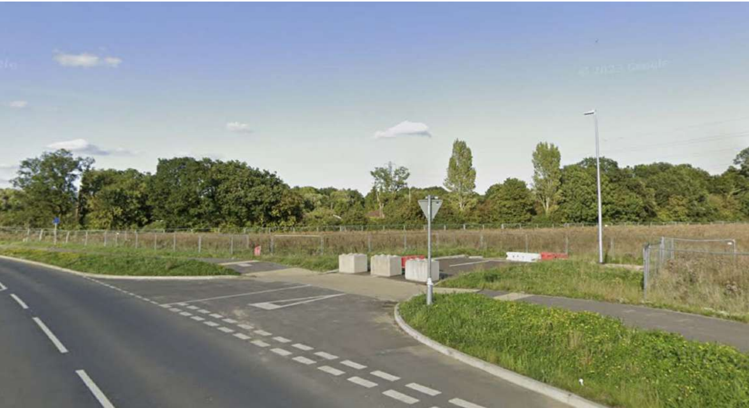
04 View from Nine Mile Ride Extension looking north-east at the newly created site access to Parcel 13
