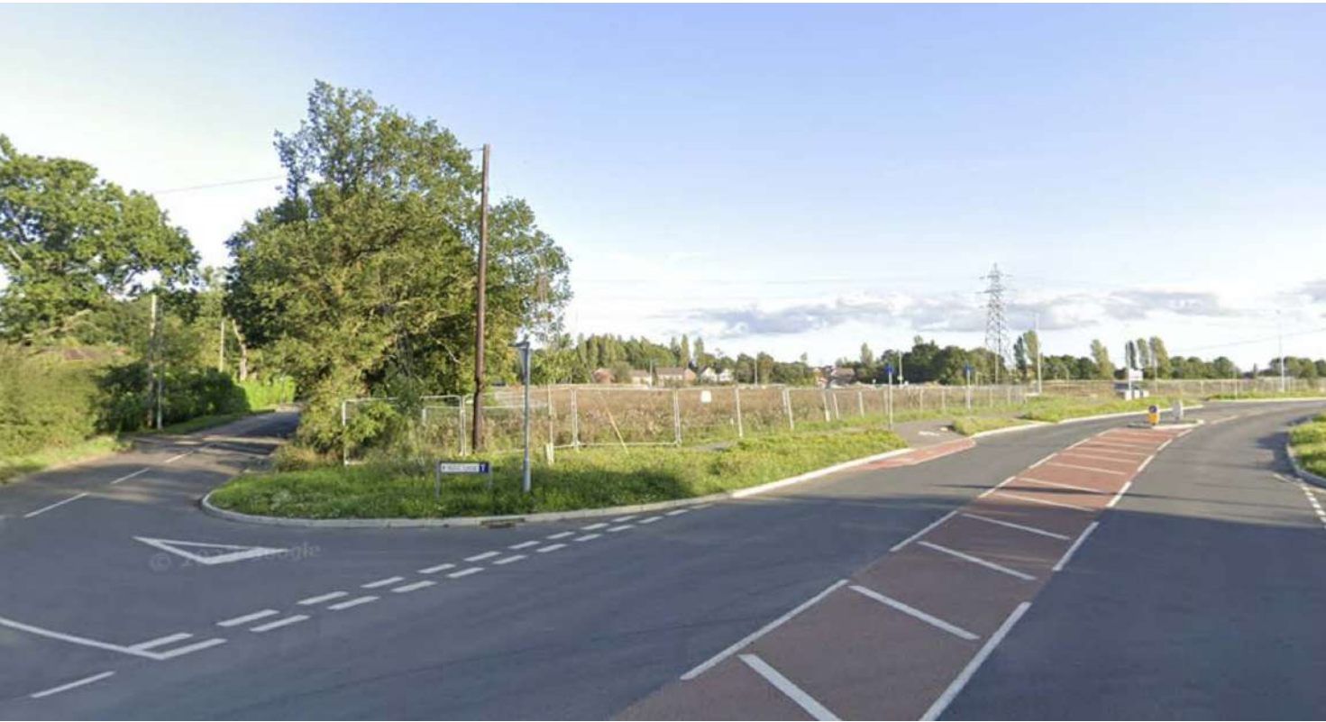
02 View from the junction with Park Lane in the north-west corner of Parcel 13, looking south-east
