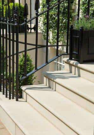
(4) Stone Steps with Metal Balustrading
