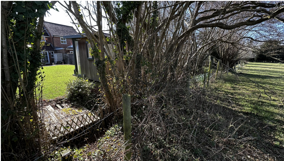
Photograph 3: Structure over waterway
