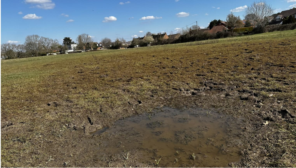
Photograph 5: Ponding at eastern side of site
