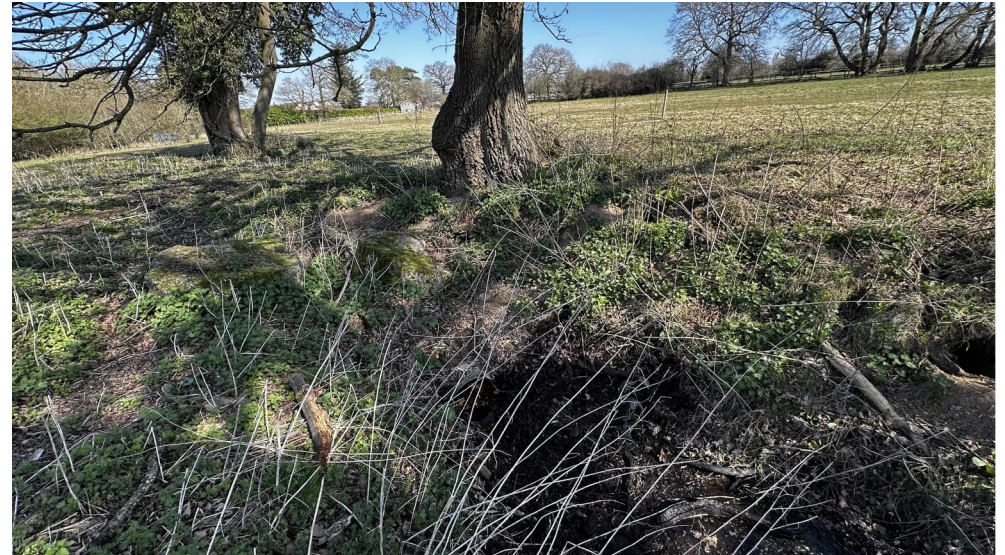
Photograph 4: Culvert in northern direction
