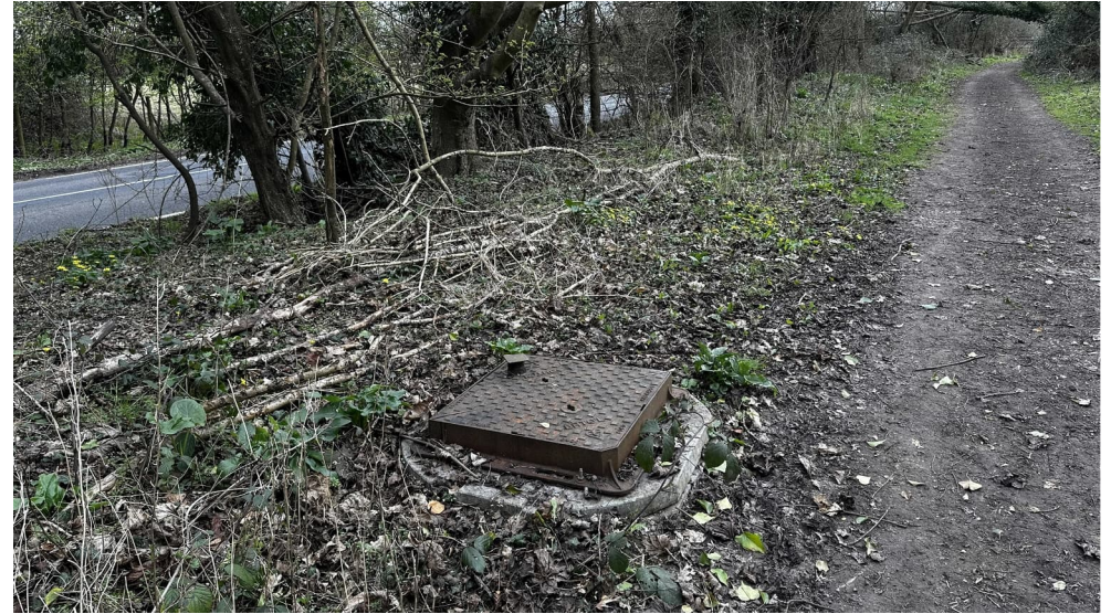
Photograph 10: Manhole in a northeastern direction from site
