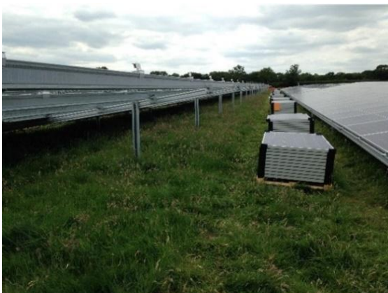
Examples of solar panels stacked ready for installation onto framework.
