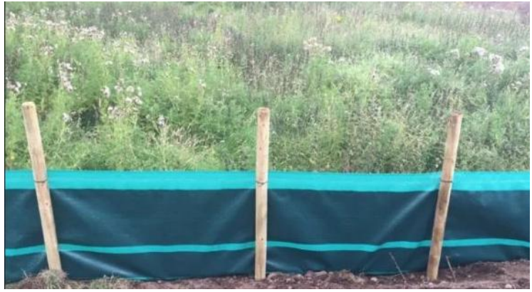
Example of silt fence/amphibian/reptile barrier to be installed alongside H11 and at the base of the security fence along the south boundary.
