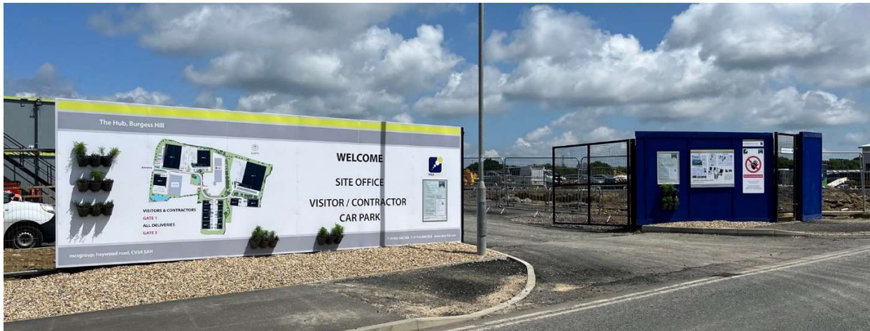
Example of typical mcs site entrance hoarding
