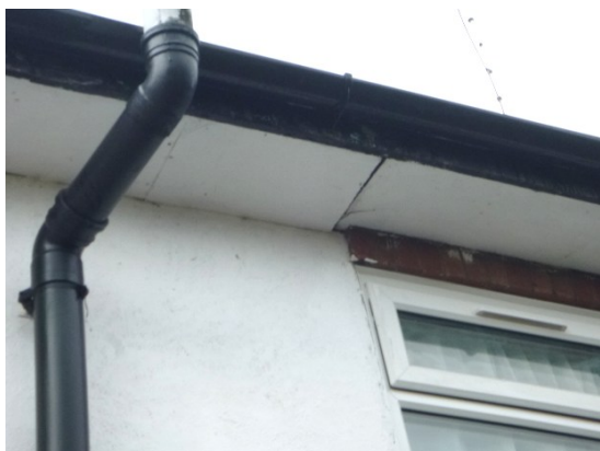
7. Separating soffit boards (rear elevation).
