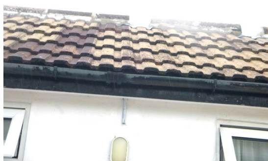
11. Large flat concrete roof tiles on single-storey extension (front elevation).
