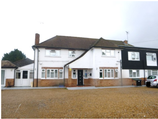
1. Front of property viewed from south.
