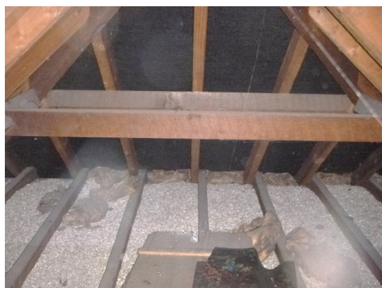
19. Eaves filled with fibreglass and paper.
