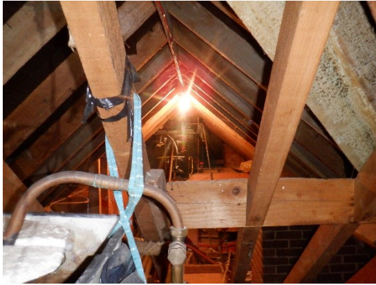
14. Roof void viewed from eastern end.
