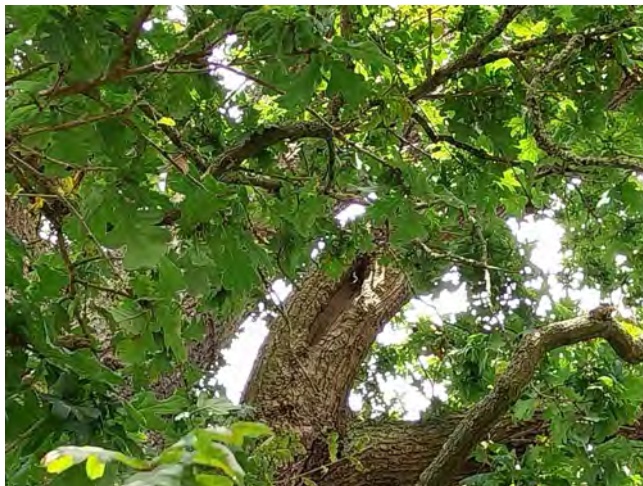
Photograph 9: A potential roost feature that is located on T1.
