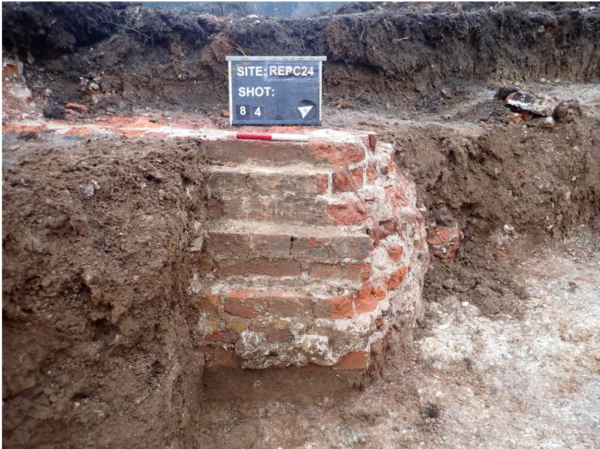
Plate 8. Foundations of garden wall (23015). Looking northwest.
