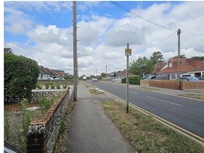
Existing highway view west
