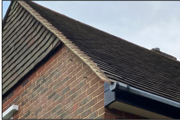
Photograph 2. Flush roof and hanging tiles on the front aspect.
