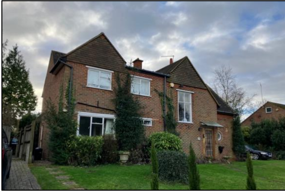
Photograph 1. The front elevation of the property.
