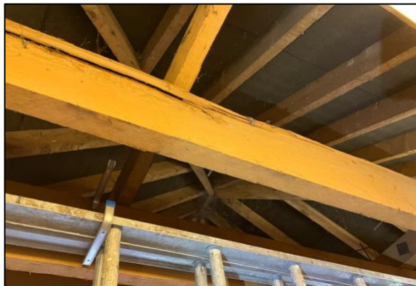
Photograph 8. Internal roof pitch of the garage.
