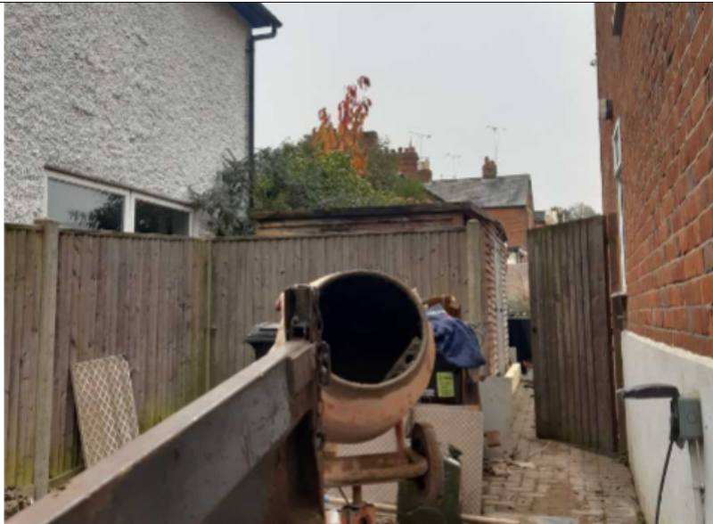
Fig 1: Image showing side facing window at no. 15A Oxford Road
