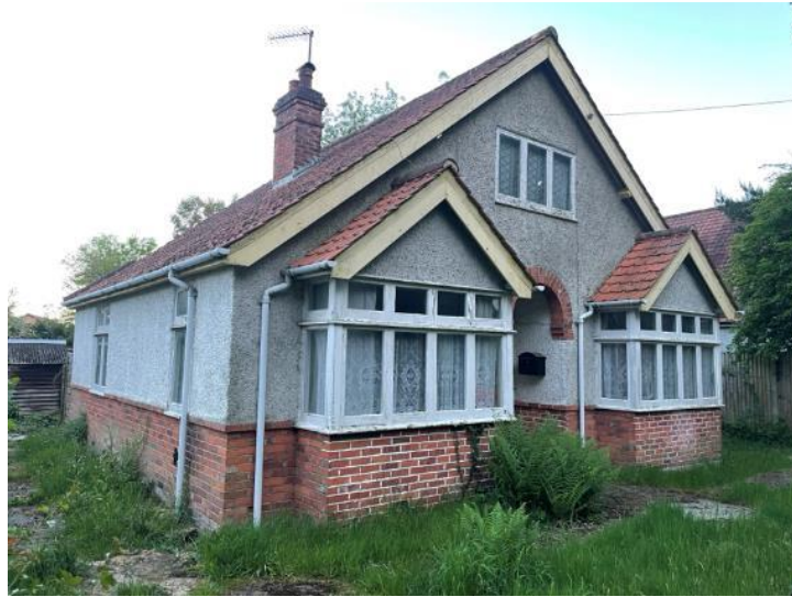
Figure 2: the northern and western elevations of B1
